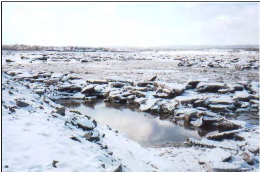
Figure 17: Temporary pool of tidal water formed along dyke near tourist bureau. Photo by D. van Proosdij, Feb. 25, 2005.
