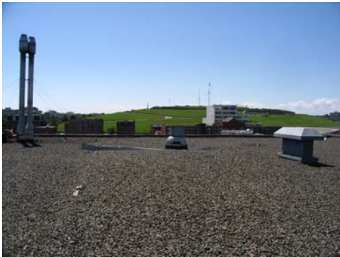
Photo 2.2; View to Citadel Hill from Joe Howe Building
