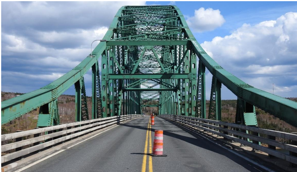
Figure 4: Seal Island Bridge at deck level
