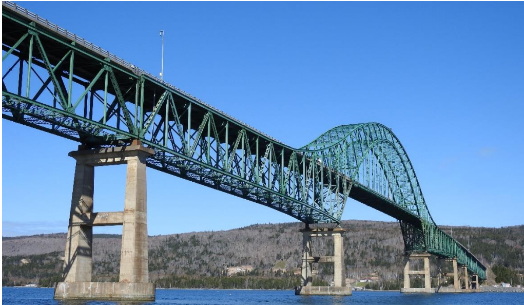
Figure 3: Seal Island Bridge north face
