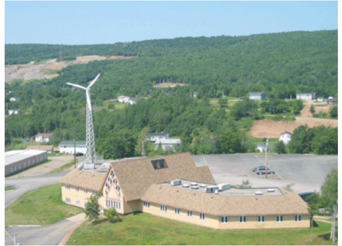
Picture 1 50kW Wind Turbine, Eskasoni First Nation, NS Courtesy of Atlantic Orient Canada Inc.
