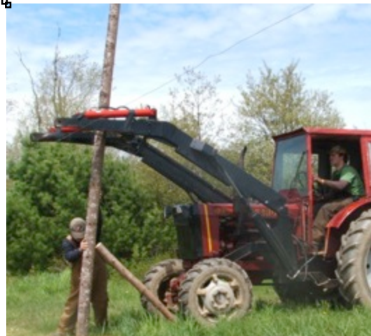
Photo 8 - Placing Trellis Poles - Courtesy of Meander River Farm
