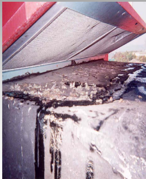
Bird Droppings at Supply Intake
