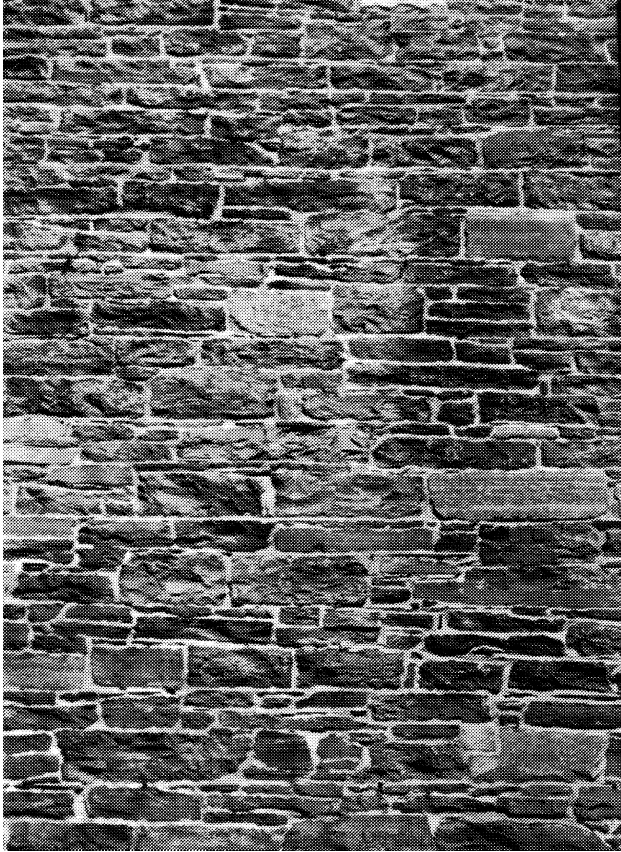
Figure 11. Wall at Historic Properties in Halifax (location 3, Fig. 7) constructed from blocks of Meguma Group slate and quartzite. The source of the material is probably similar to bedrock observed in Figure 10.
