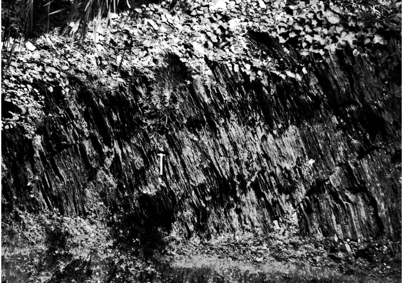
Figure 24. This recently exposed slate road cut at Waldeck, Annapolis County (location 9, Fig. 7b), demonstrates how quickly weathering can take place. Rubble at the base of this outcrop is the result of weathering.
