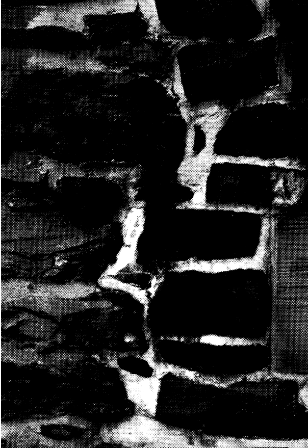
Figure 18. Iron stained (dark blebs and stains in white) mortar resulting from exposed pyrite in a slate wall, downtown Halifax (location 3, Fig. 7). Just one or two pyrite crystals in the rock can ruin the visual appeal of a structure.
