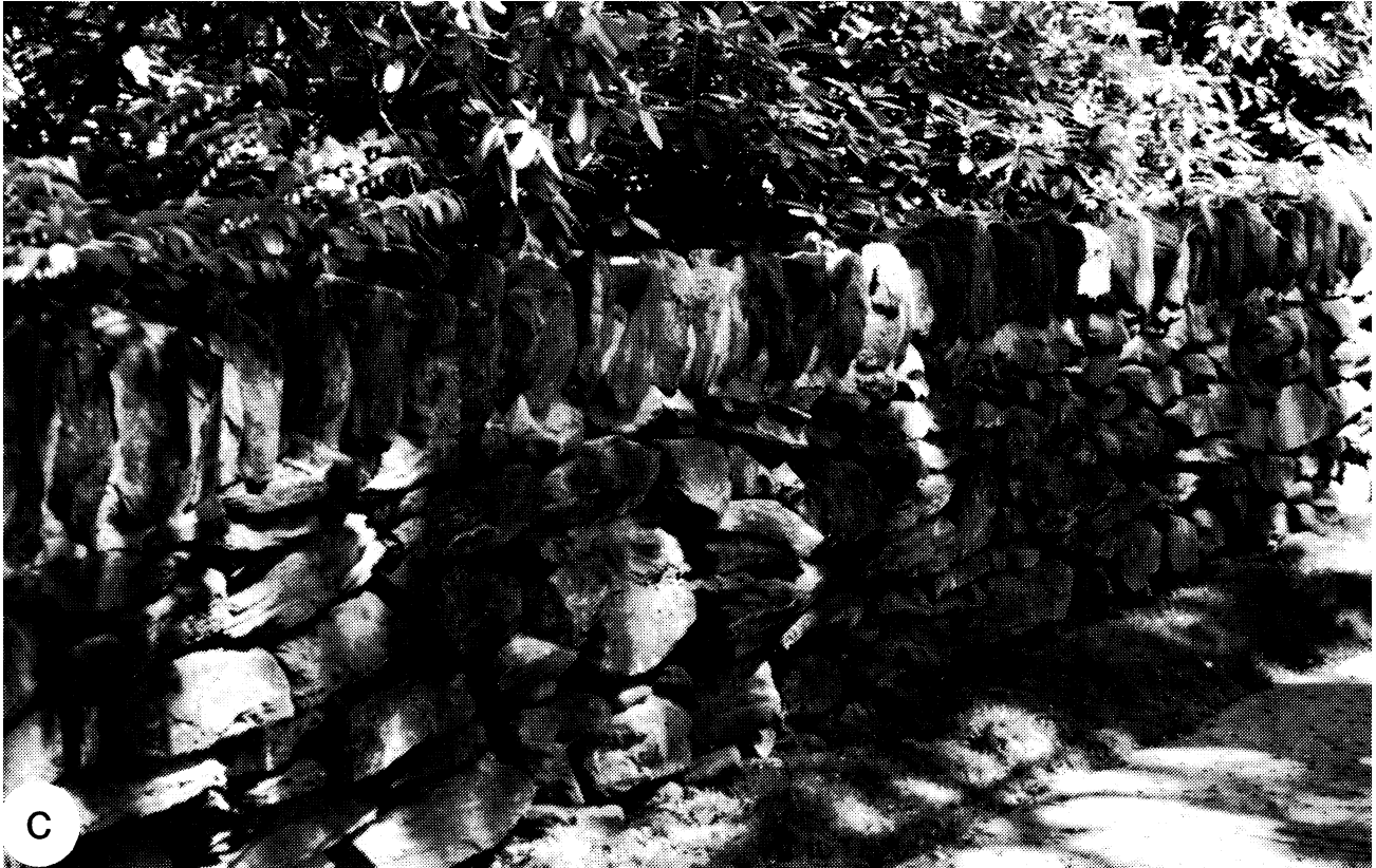
Figure 17. Examples of quartzite and slate dimension stone in the Metro area. (a) This stone building in Point Pleasant Park (location 6, Fig. 7) is a testimony to the lasting architectural appeal of quartzite as a building stone. (b) Retaining walls constructed of quartzite are a common site in Metro. The mortared wall shown here is in Rockingham (location 7, Fig. 7). (c) Fence rows of slate are a focal point in the south end of Halifax (location 8, Fig. 7).
