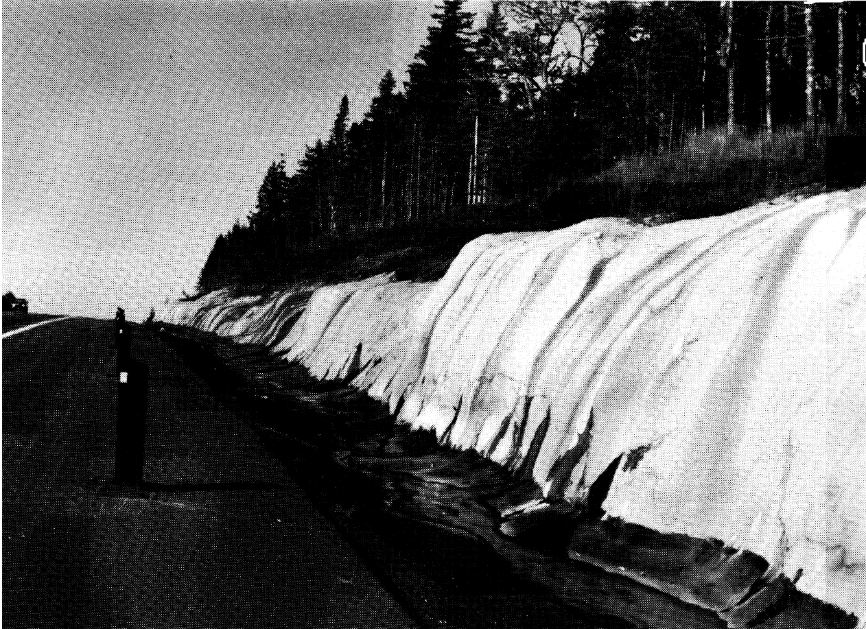
Figure 16. Attempts to seal acid-generating slates exposed during construction of Route 107 near Petpeswick Lake (location 5, Fig. 7) have not eliminated the problem. Rusty, iron stains (they look like shadows in the photo above) on the shotcrete and in the drainage ditch are a telltale sign of acid-generating slate. A containment pond at the base of this hill is used to buffer the low pH runoff before it enters the local lake system.
