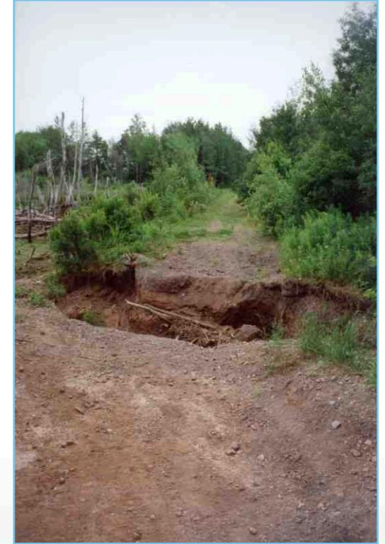
Road erosion is a common problem, and can lead to road surface deterioration, silted streams and other runoff problems. Proper ditching technique and shaping and crowning the road can prevent future drainage problems. If possible, roads should be constructed on slight slopes to help the water to move away from the road surface.
