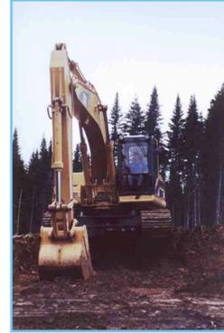
After the right-of-way is cut and the wood removed, the road is ready to be built. Excavators are effective in digging ditches and using the soil material to construct the road bed. Bulldozers can also be used, although some areas adjacent to the road will need to be cleared for push-offs.
