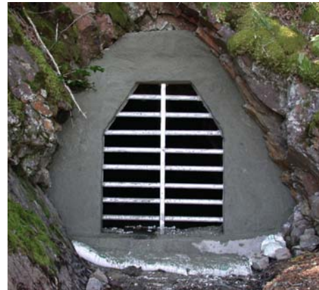
Figure 2. Mine opening after the closure project.
