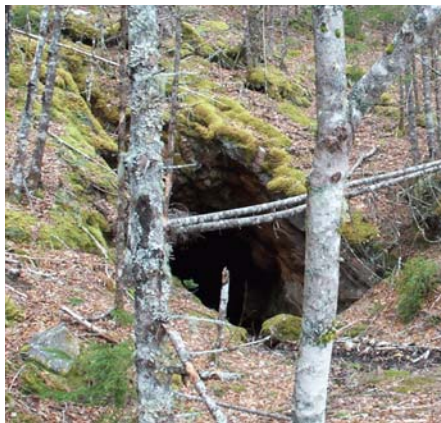
Figure 1. Mine opening at Lake Charlotte before remediation.
