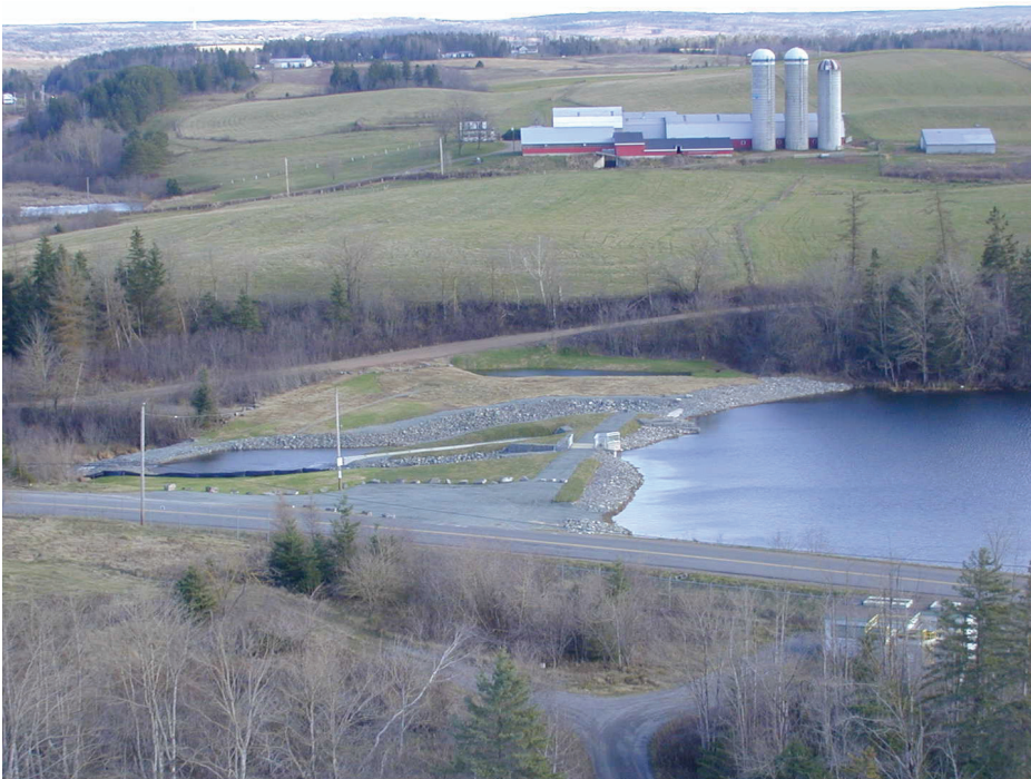
Figure 1. View of the refurbished Shortts Lake Dam.
