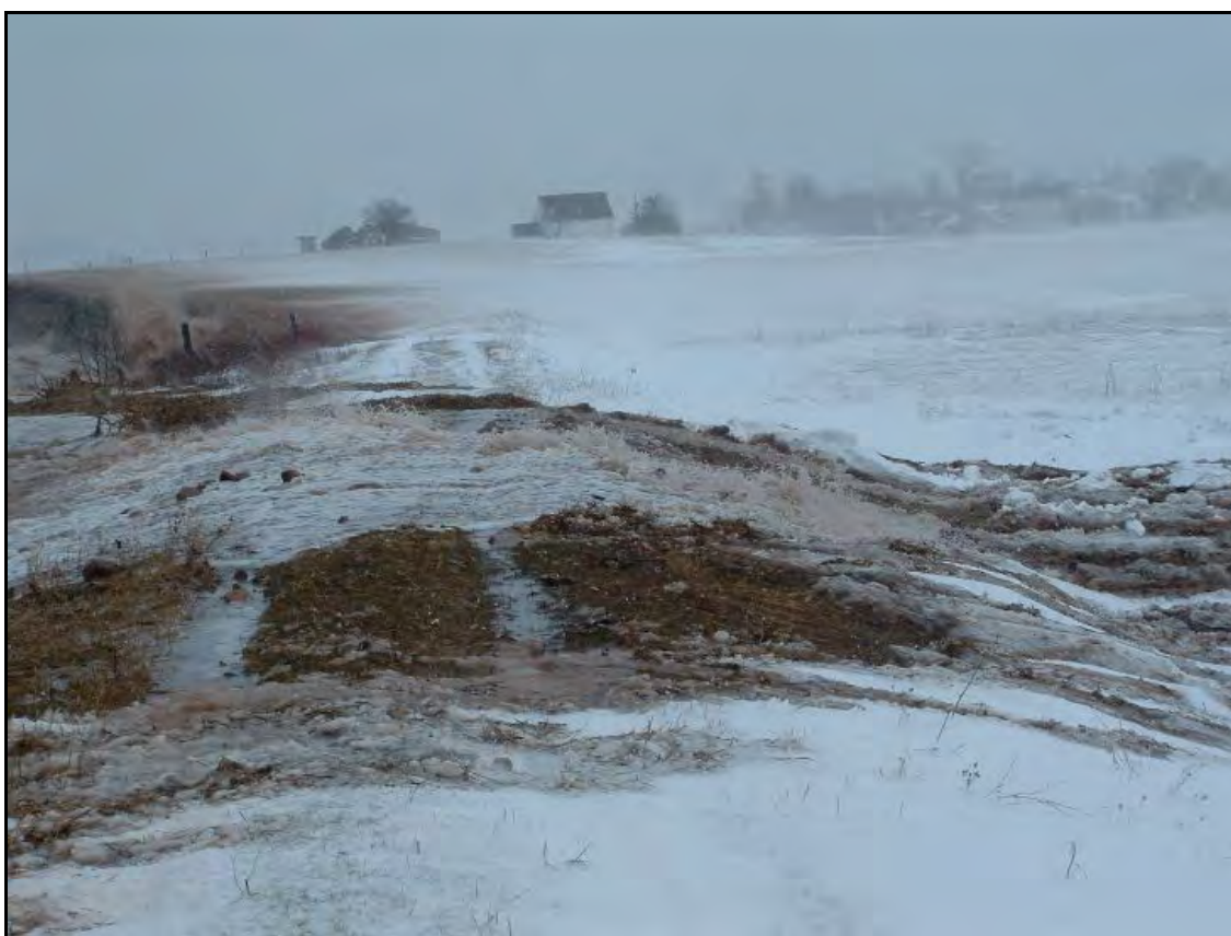
Figure 26: Storm impacts on Feb 1, 2006 at the Avonport Dyke. a) storm waves battering marsh; b) storm surge reached upper limits of dyke and c) dyke overtopped. Photo by T. Hamilton, 2006.
