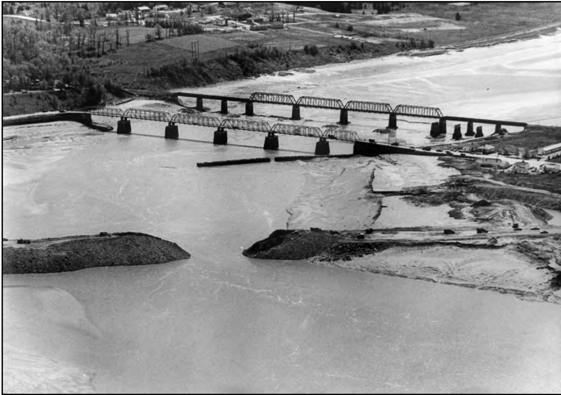
Figure 9: Final phase of the construction of the Windsor Causeway, around November, 1969. Photo from NSDA archives. Note presence of groyne installed during the construction process.
