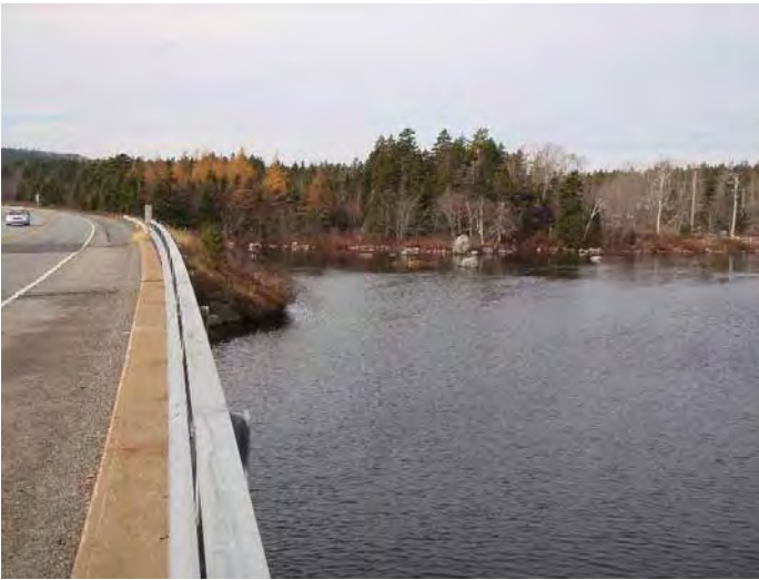
Watercourse 6: Mill Lake – West Shoreline
