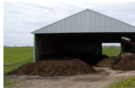
Fig. 3 Compost pile ready to sample
