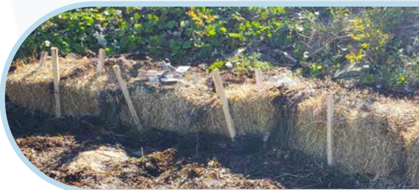
Straw bale soft armouring example
