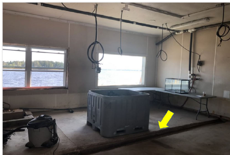
Figure 6. Existing water discharge grate outflow pipe runs below plant
