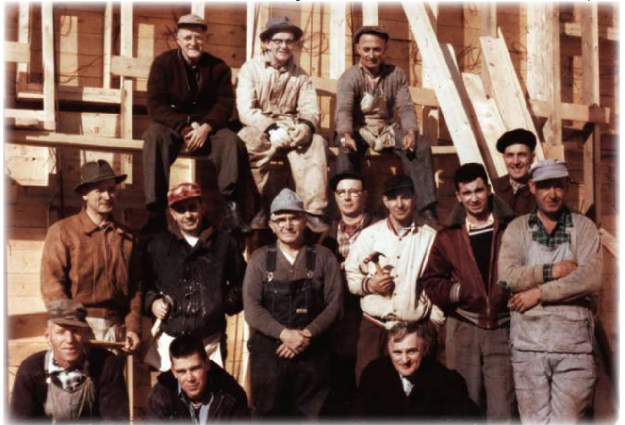
The construction of Stairs Memorial United Church on Hester Street in the late 1950s was a community project that drew parishioners together and inspired a spiritual renewal in Dartmouth North.
