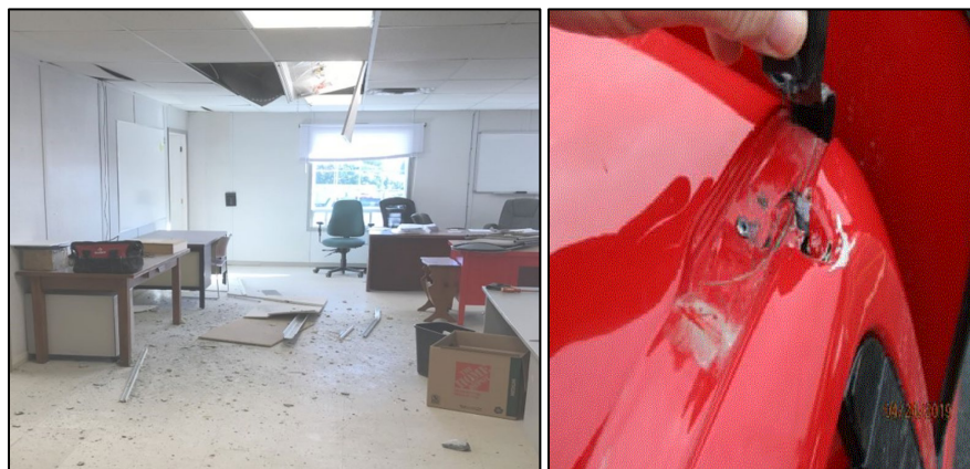
Figure 1 – Flying material damage to a site trailer and a parked truck from two separate blasting incidents.
