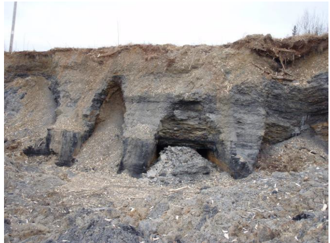
A sideview of a bootleg coal site, which represents a potential geohazard.
