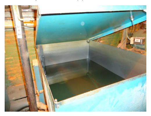
Photo 4: Hydraulic reserve tank, in the basement beneath paper drying machines.
