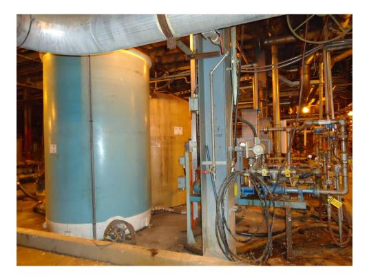
Photo 10: Primary and secondary retention aid tanks
