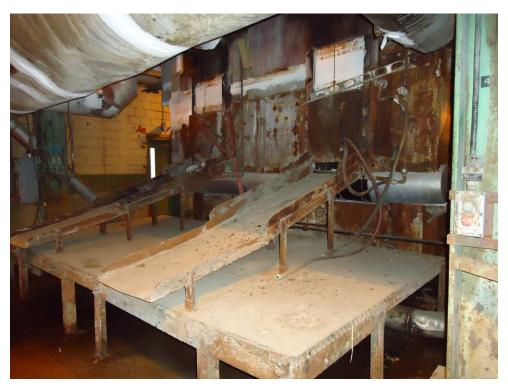
Photo 13: Boiler 4, was powered by bark and bunker C.
