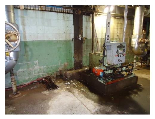
Photo 12: Small oil reserve and staining present within the basement of the paper processing area.
