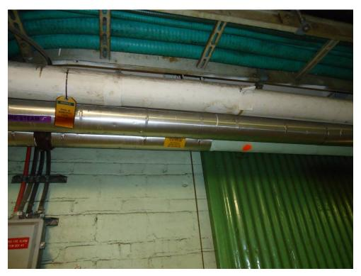
Photo 11: Piping labelled within plant as asbestos containing in the background, and none asbestos containing in the front.
