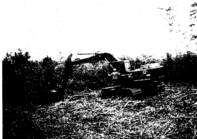
Figure 1. The Denis-Cimaf TRH-150 Brush-Cutter in site clearing.
