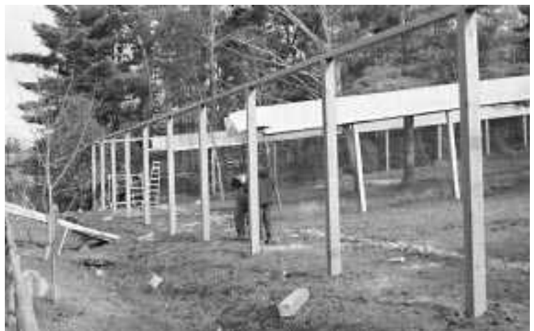
Rebuilding hurricane damaged enclosures for Wildlife Park residents.
