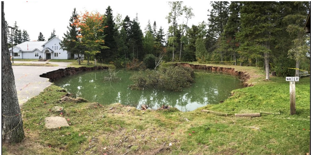
Figure 2. Photograph of the sinkhole in September 2018.
