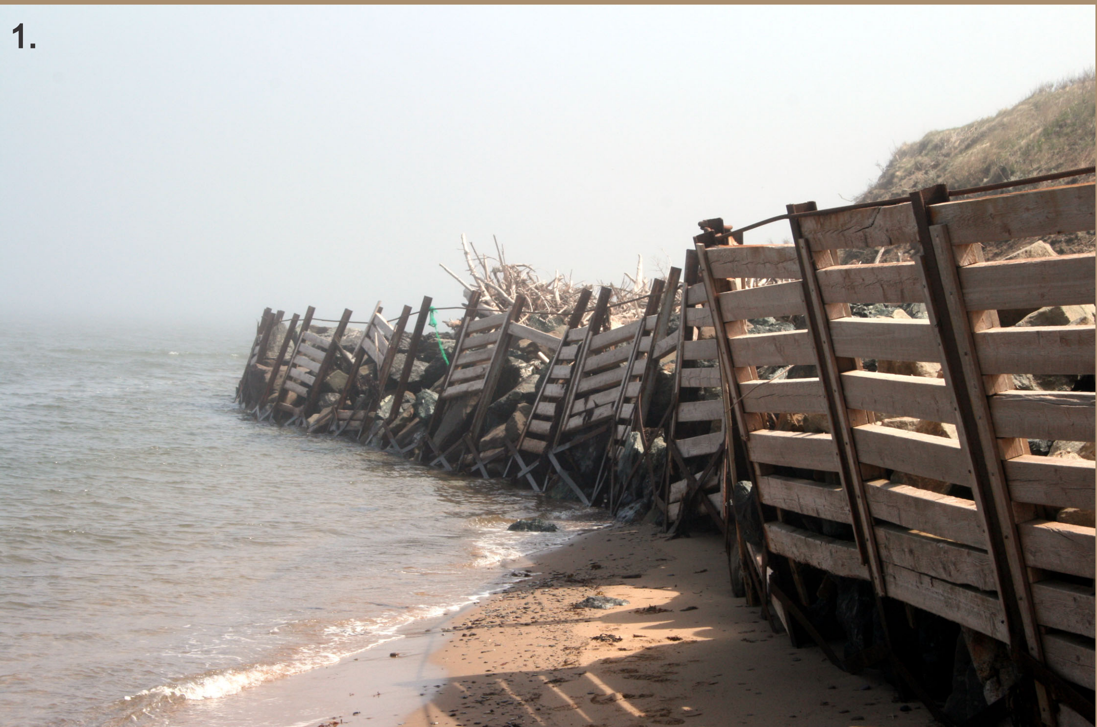
Figure 1. Inadequate understanding of coastal processes and a lack of knowledge of the underlying bedrock geology has resulted in the rapid collapse of this engineered structure.
