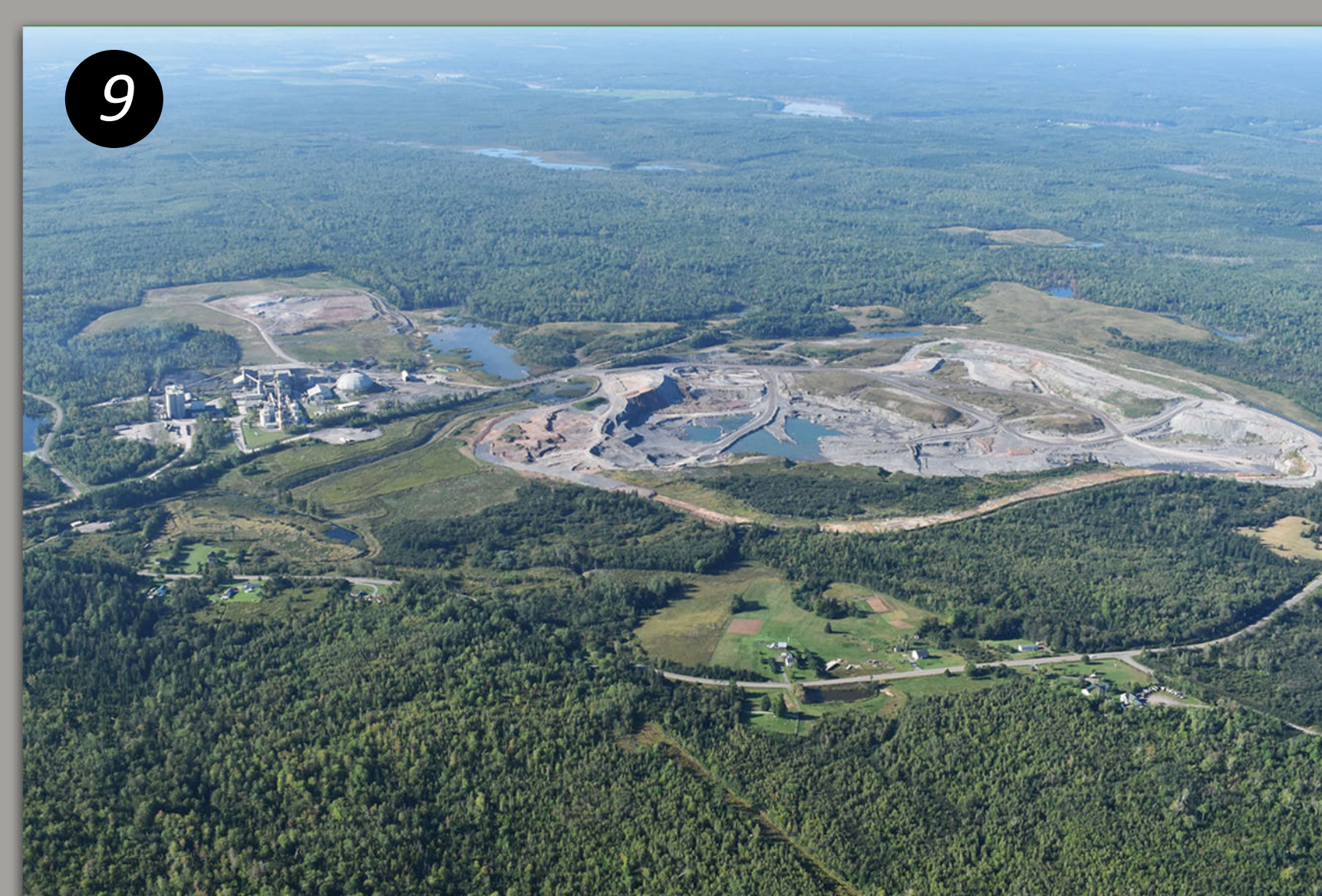
9 Lafarge Canada Inc. Brookfield - limestone
