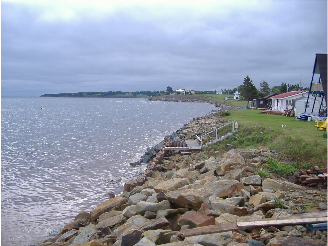
Figure 2. Extensive armouring along the coastline.
