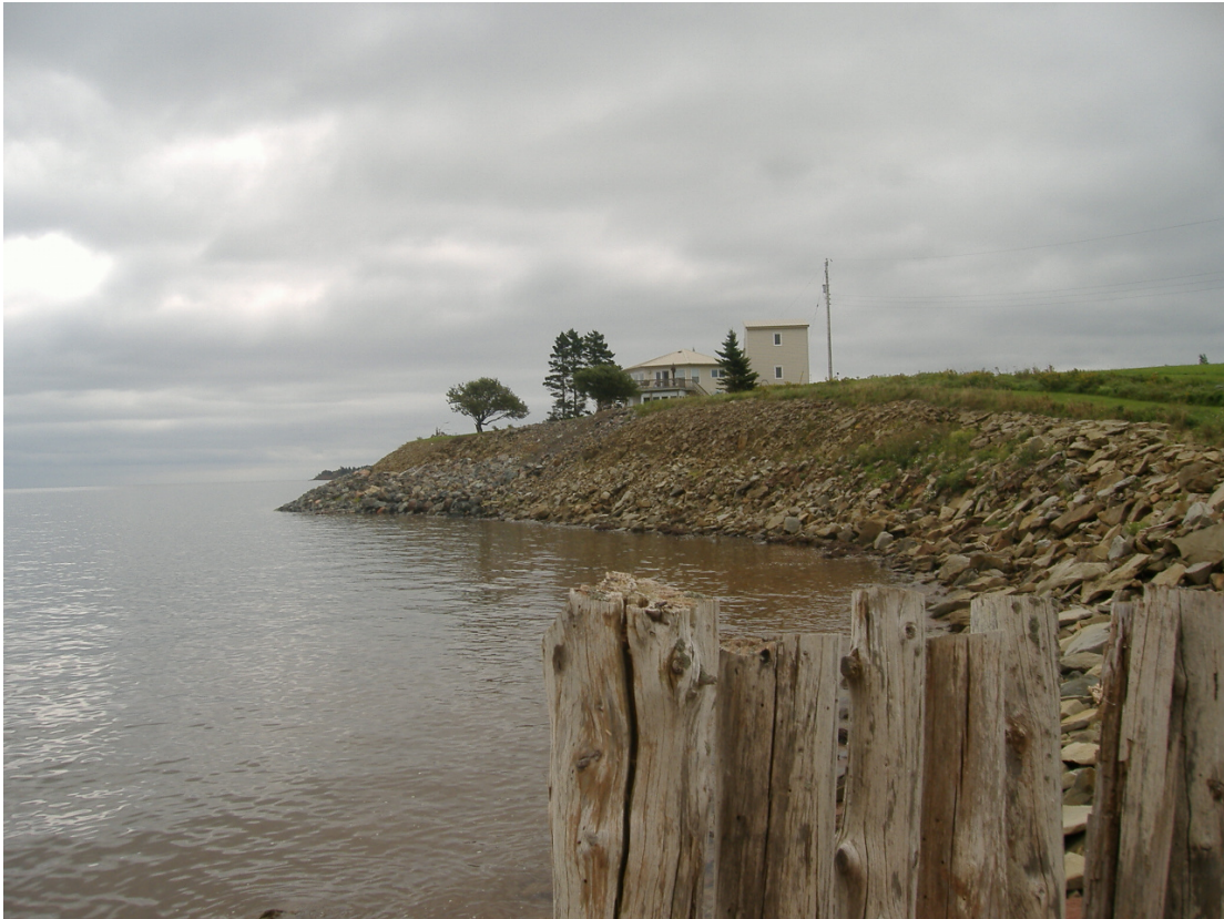
Figure 7. Retaining wall constructed by simply dumping stone over the bank.
