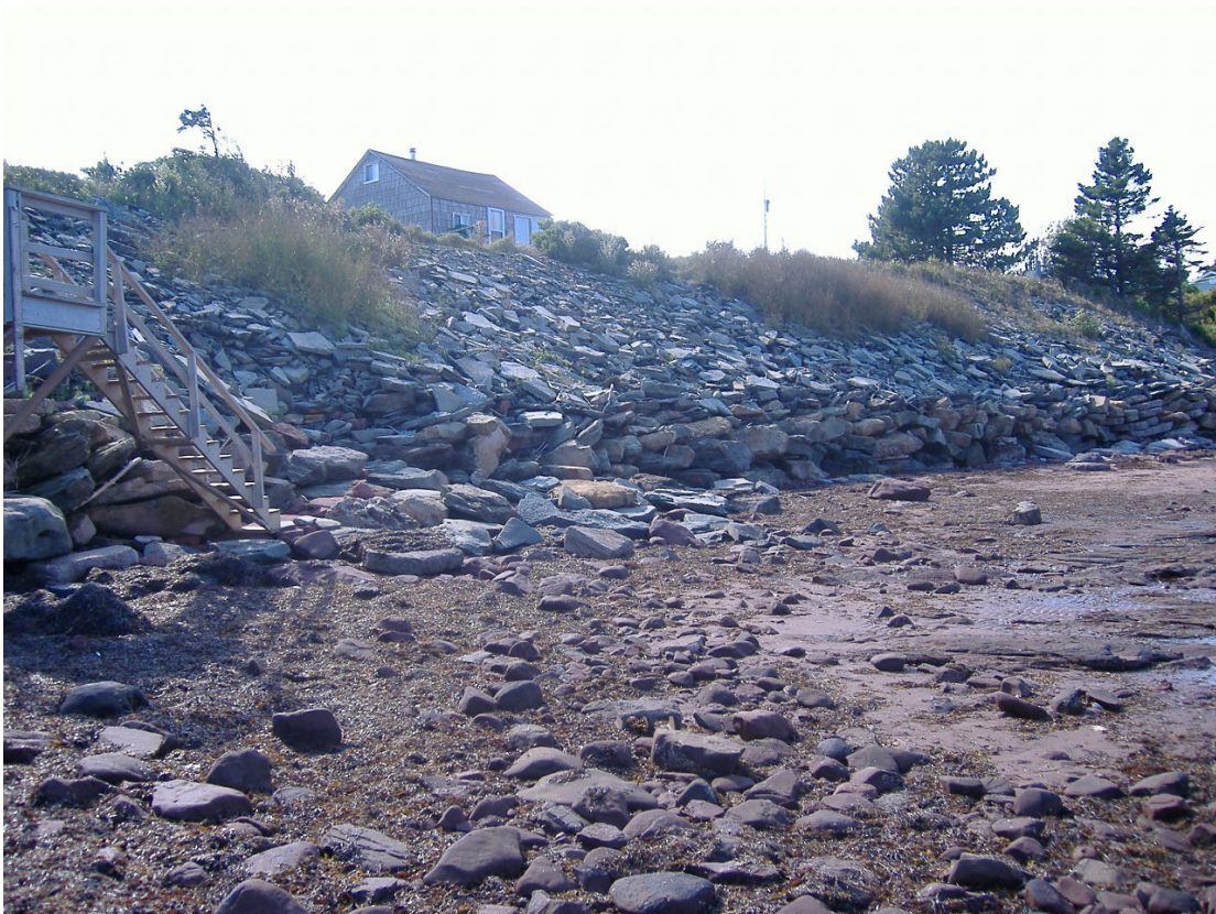
Figure 8. Retaining wall illustrating stone placement at base with dumping of stone along upper bank.
