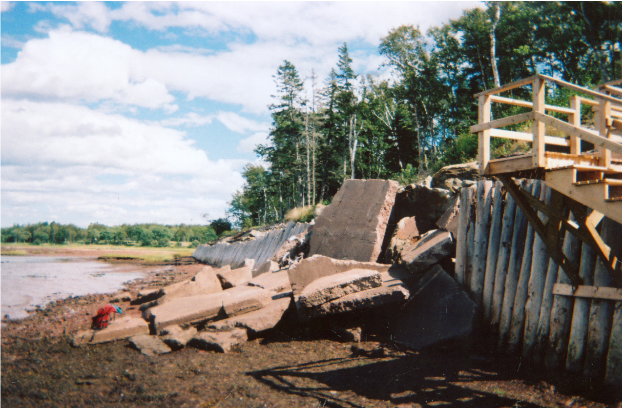
Figure 4. Slabs of concrete construction waste used for coastal hardening.
