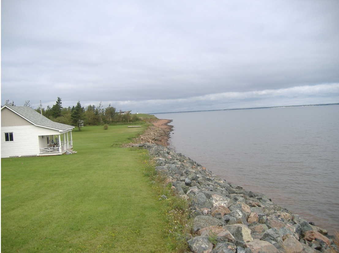
Figure 9. A retaining wall with reasonably placed armour stone.
