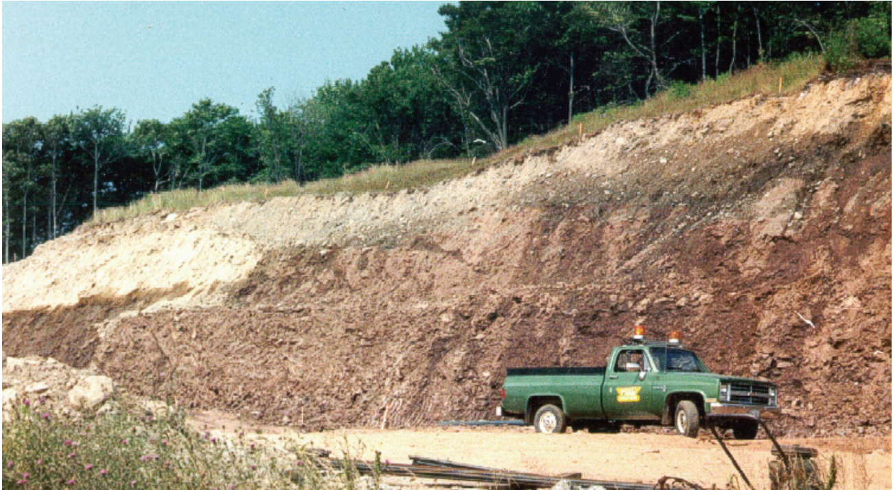
Figure 7. Photograph of Lawrencetown Till overlain by Beaver River Till excavated during construction of the MicMac Parco overpasses in the early 1990s in Dartmouth to replace the former MicMac Rotary. Photograph courtesy of R. Stea.
