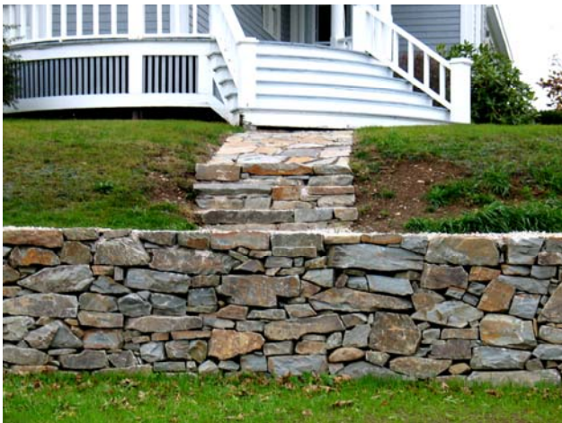
Figure 8. This stone wall and steps were constructed from joint-fractured metasandstone and are another example of the quality of work done by stone masons. Selecting pieces from the pile that will fit the wall with minimal trimming requires an experienced eye for stone.
