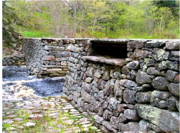
Figure 7. This dam at Gardners Mills, Yarmouth County, is constructed of Goldenville Group metasandstone, which was most likely obtained from fieldstone (glacial till boulders). It is an excellent example of the skill that goes into the construction of these structures.
