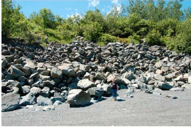
Figure 14. Armouring at base of the Rail Line Slide. Photo location is at Site 5 on Figure 12.
