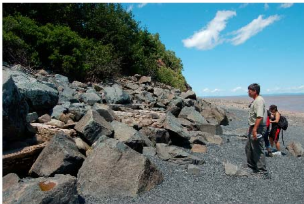
Figure 15. Armour stone and wood crib work at the base of the Rail Line Slide. Location is just north of Site 4 shown on Figure 12.
