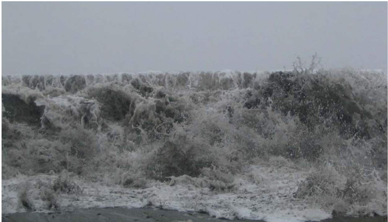
Figure 8. Water overtopping the Gabarus seawall due to wave run-up.
