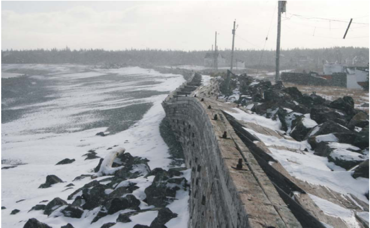
Figure 15. Severe deterioration of the Gabarus seawall.
