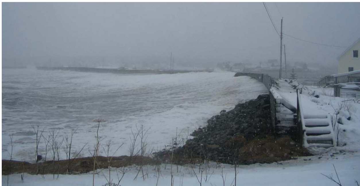
Figure 11. Wave run-up on the sediment buildup at the north end of the Gabarus seawall, with resulting overtopping and flooding behind the seawall.
