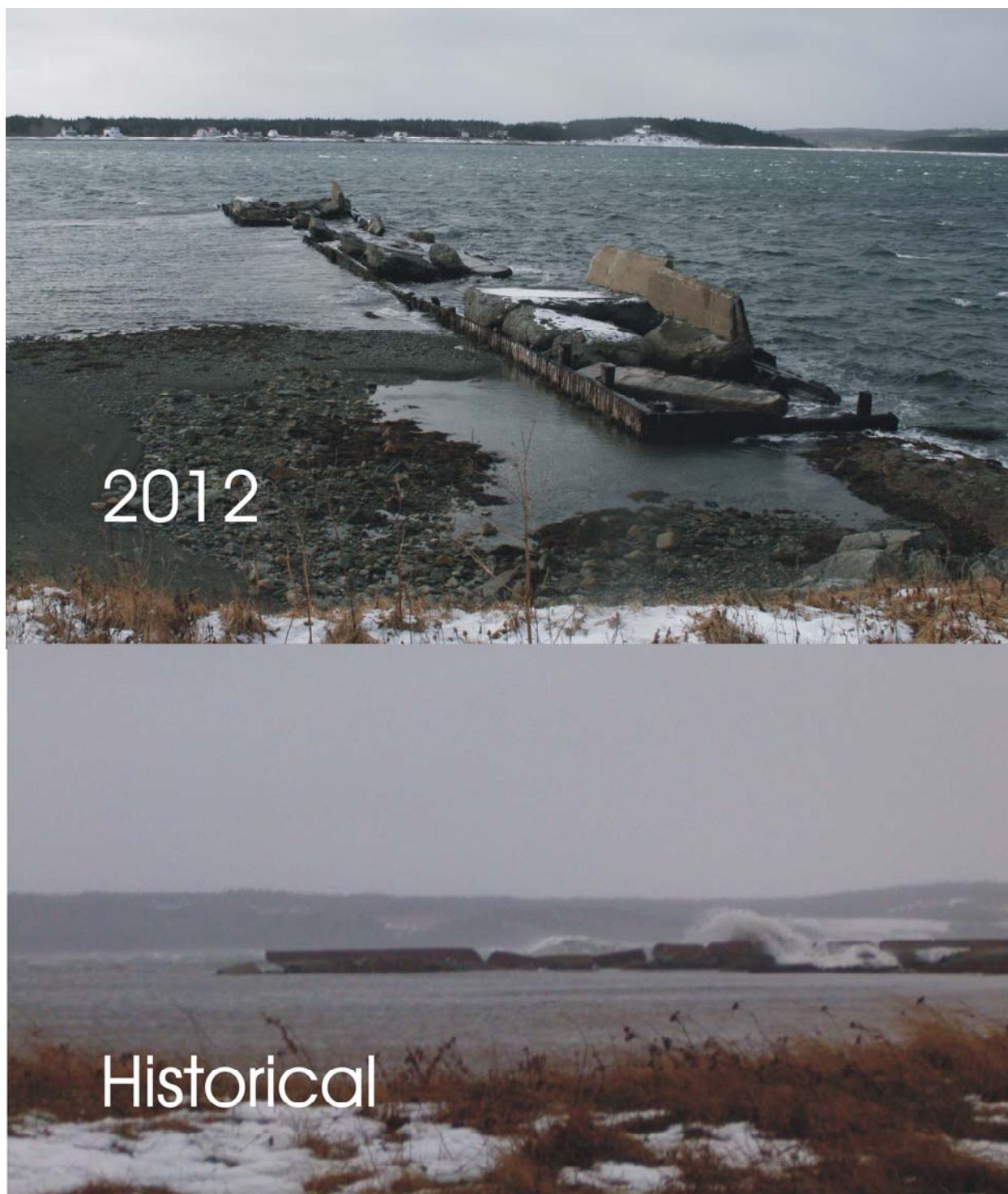
Figure 13. Historical concrete breakwater showing deterioration (bottom) with present day enhanced deterioration (top).
