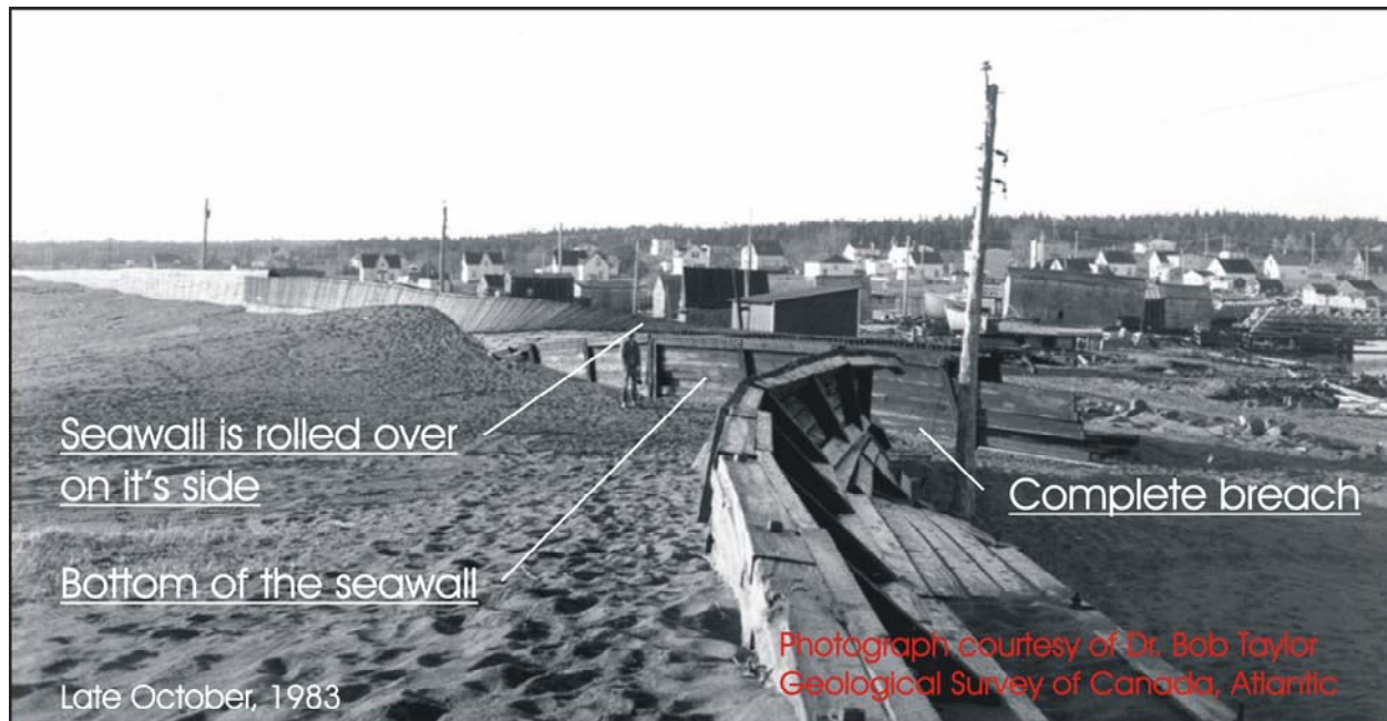
Figure 14. 1983 photograph of damage to the seawall at Gabarus. Photo by Bob Taylor, GSC Atlantic.
