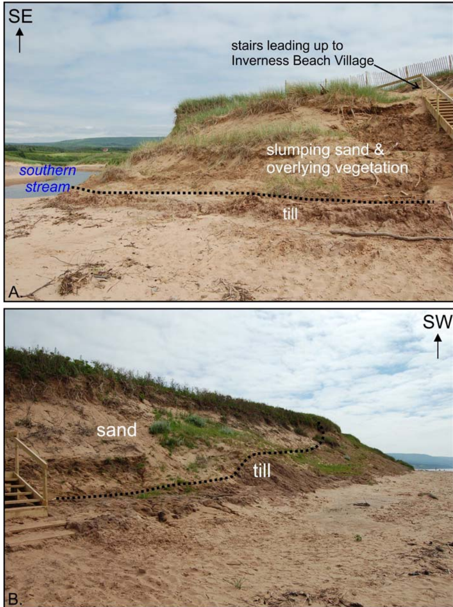
Figure 3. A) Looking southeast at silty till underlying slumping dune-sand and fluvially re-worked dune-sand. Southern stream in local valley on left side of photo and stairs leading up to Inverness Beach Village on the right. B) Looking southwest down the coast at dune sand pinching out and giving way to silty-till plain exposed in coastal cliffs.
