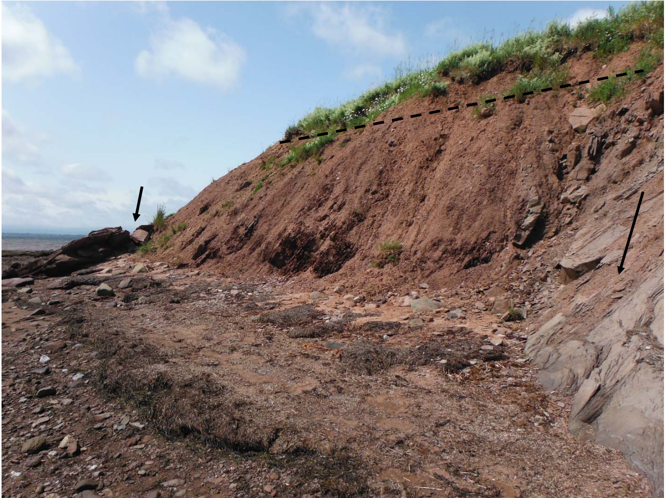
Figure 2. A shoreline image taken from the beach at Malagash Point. Note the dipping reddish-brown sedimentary beds between the two grey sandstone beds (black arrows). Only the top ~1 m of the cliff (above dashed line) is till.
