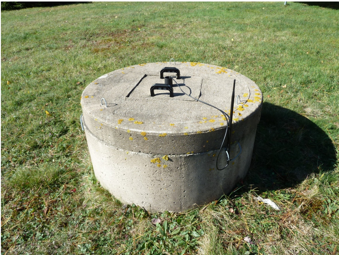
Figure 8. External antenna mounted on side of well with cable leading to meter inside well.
