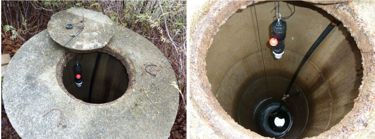
Figure 7. Water level meter installed in a dug well.
