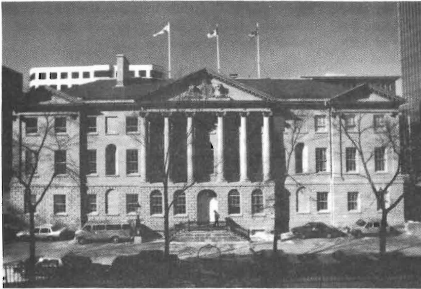
Figure A3-1. Province House, Halifax, Nova Scotia
