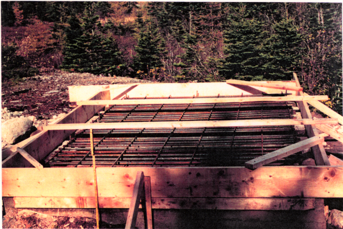
PHOTO NO. D-4: Completed concrete form with rebar reinforcement.
