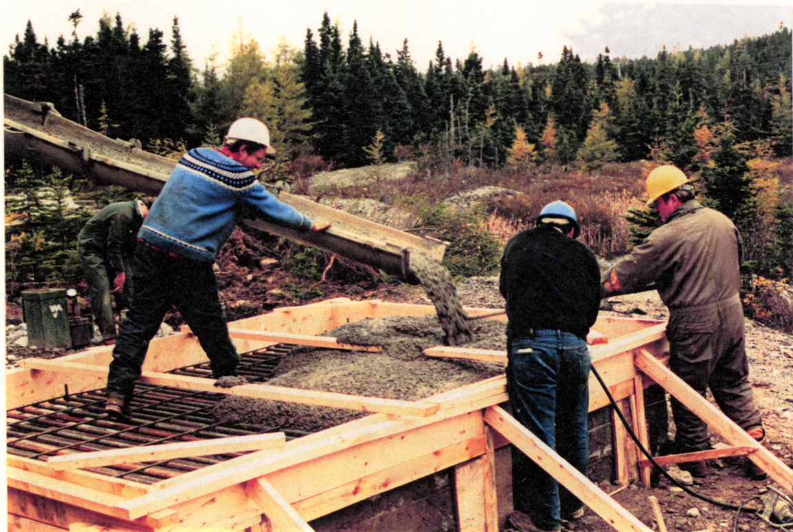
PHOTO NO. D-6: Casting concrete into form work over No. 1 Shaft.
