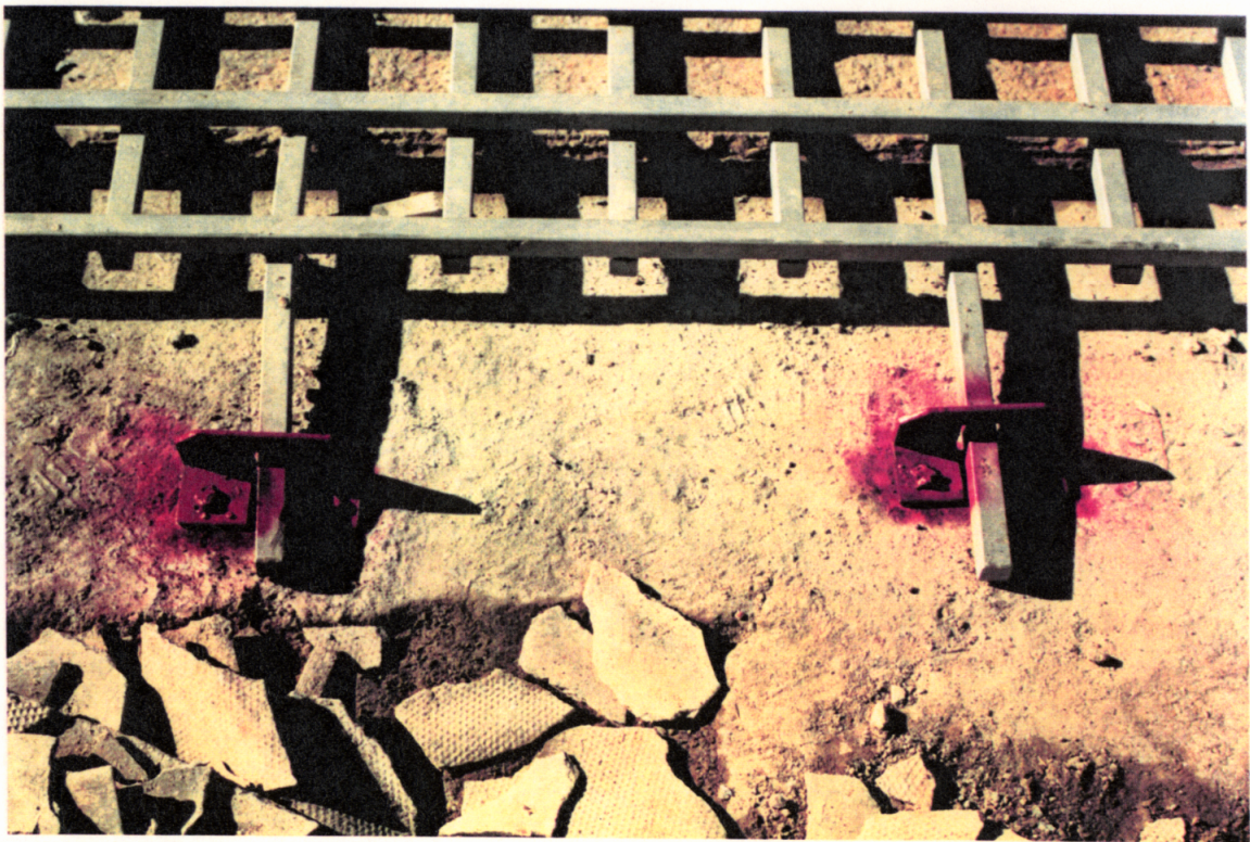
PHOTO No. E-10: Close-up of steel anchor brackets.
