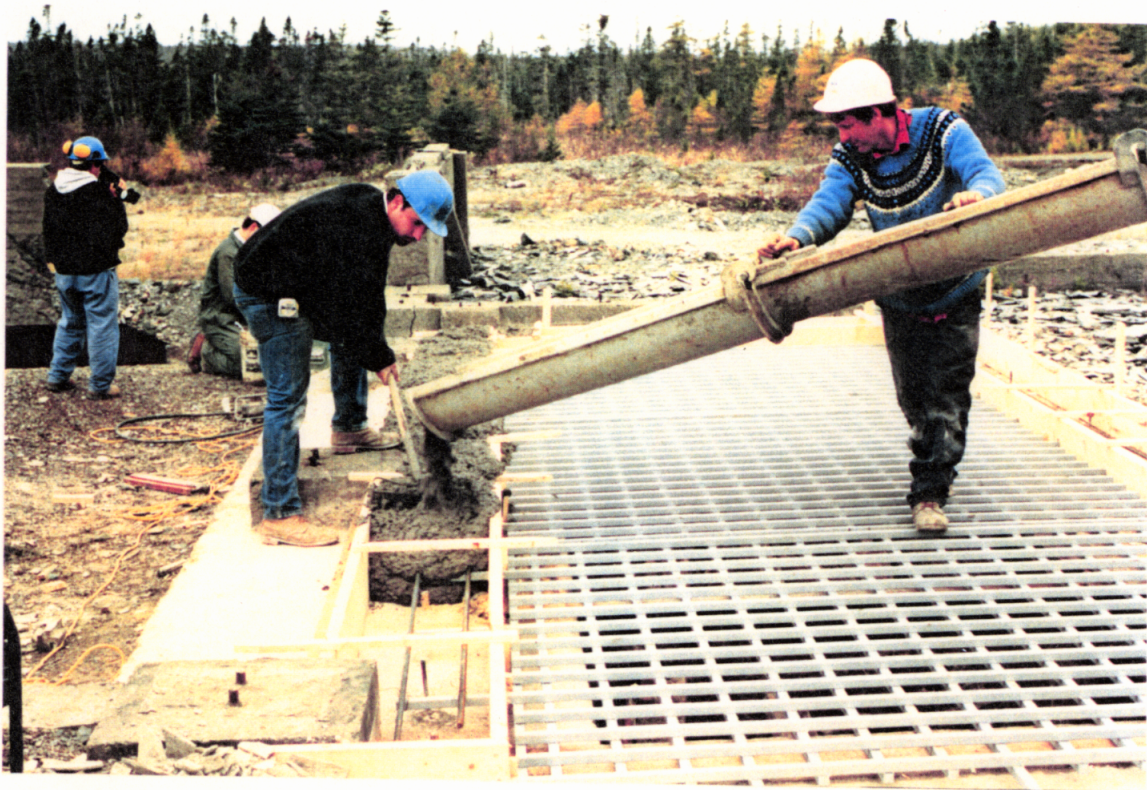
PHOTO NO. E-7: Casting concrete into collar forms showing rebar reinforcement.
