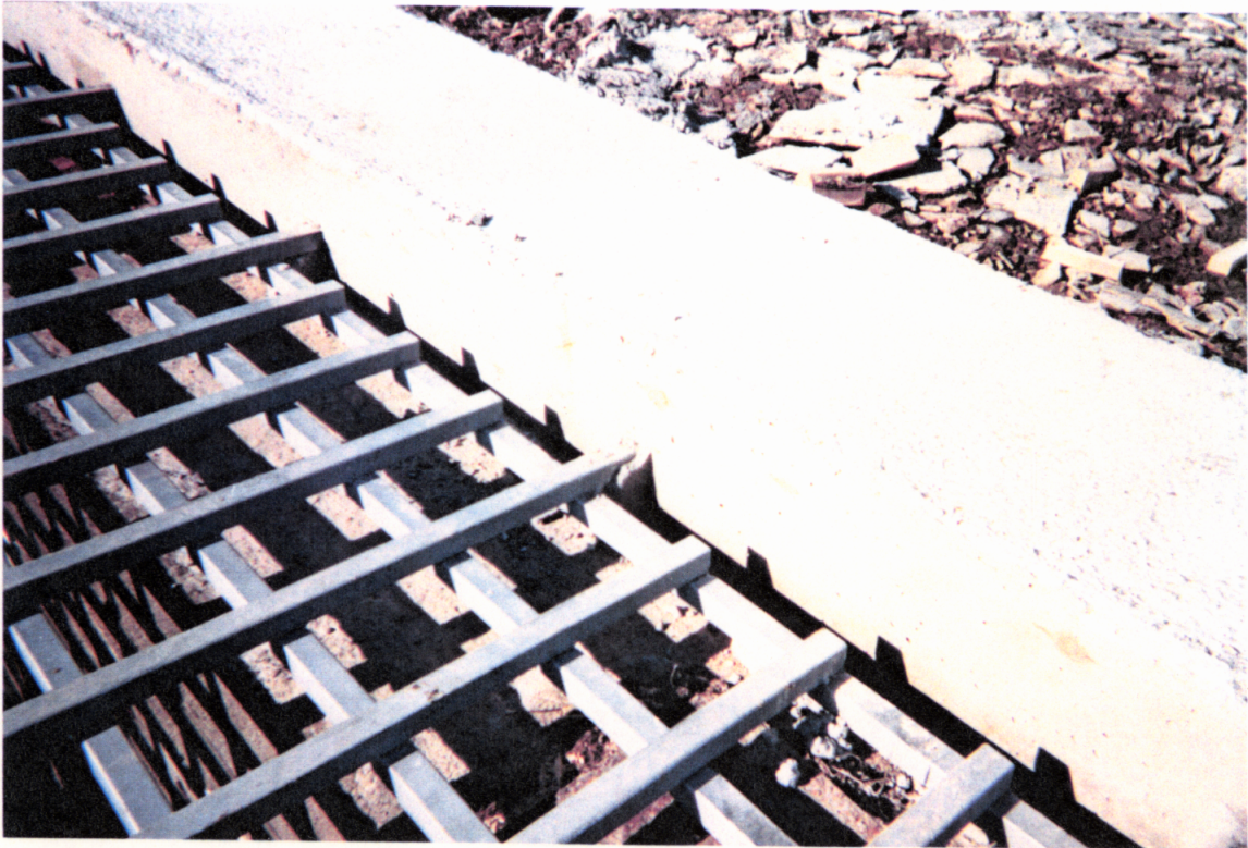
PHOTO NO. E-9: Close-up of concrete collar showing bars extending into concrete.
