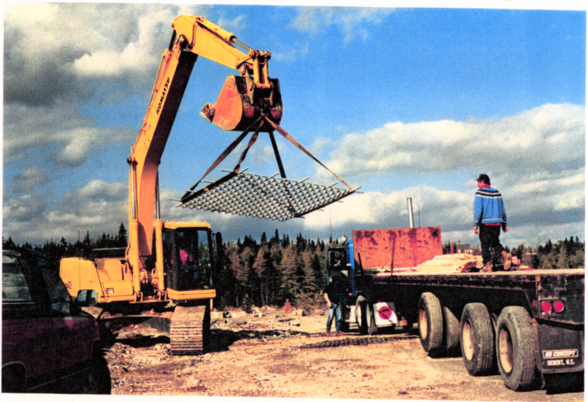
PHOTO NO. E-3: Unloading steel grating from flatbed.
