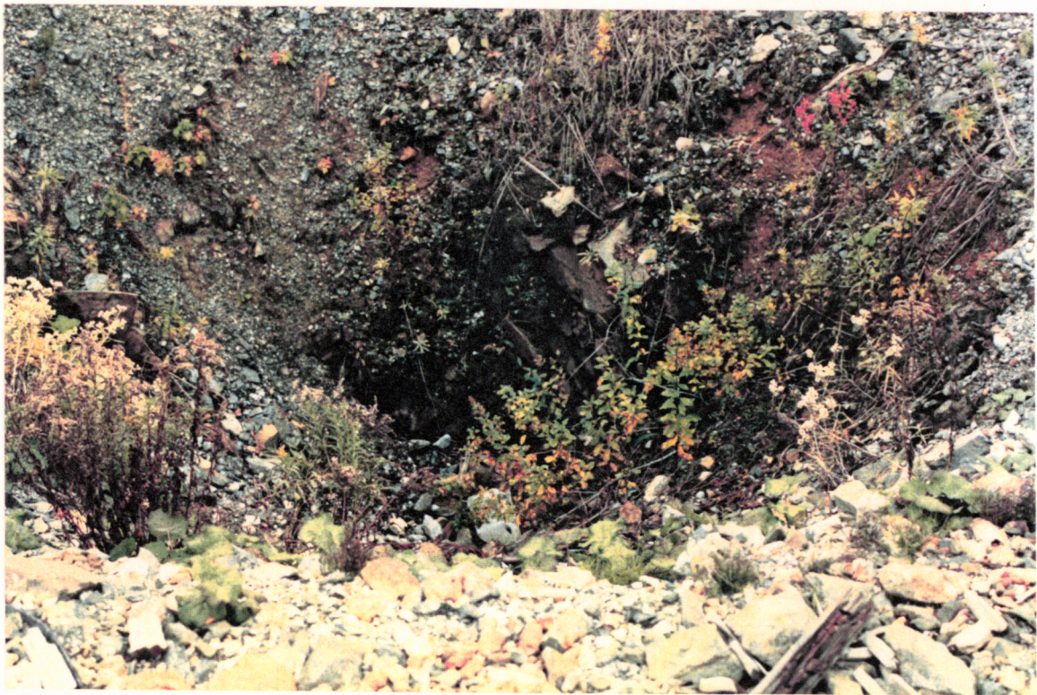
PHOTO NO. F-2: Looking into No. 1 Raise subsidence feature showing timber debris and vegetation.
