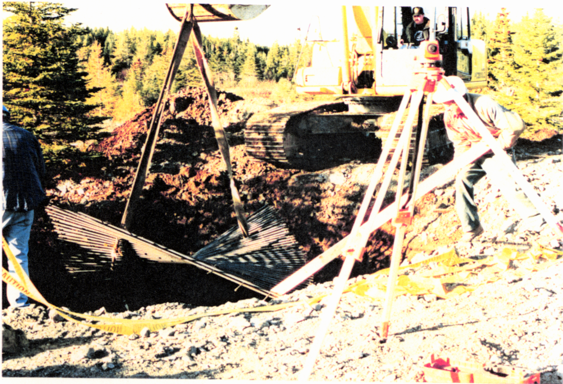
PHOTO NO. F-5: Lowering rebar reinforcing mat into No. 1 Raise excavation.
