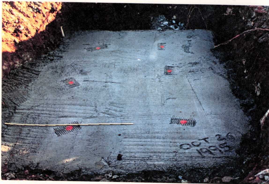
PHOTO NO. F-8: Completed concrete monolithic slab showing locations where thickness was measured.
