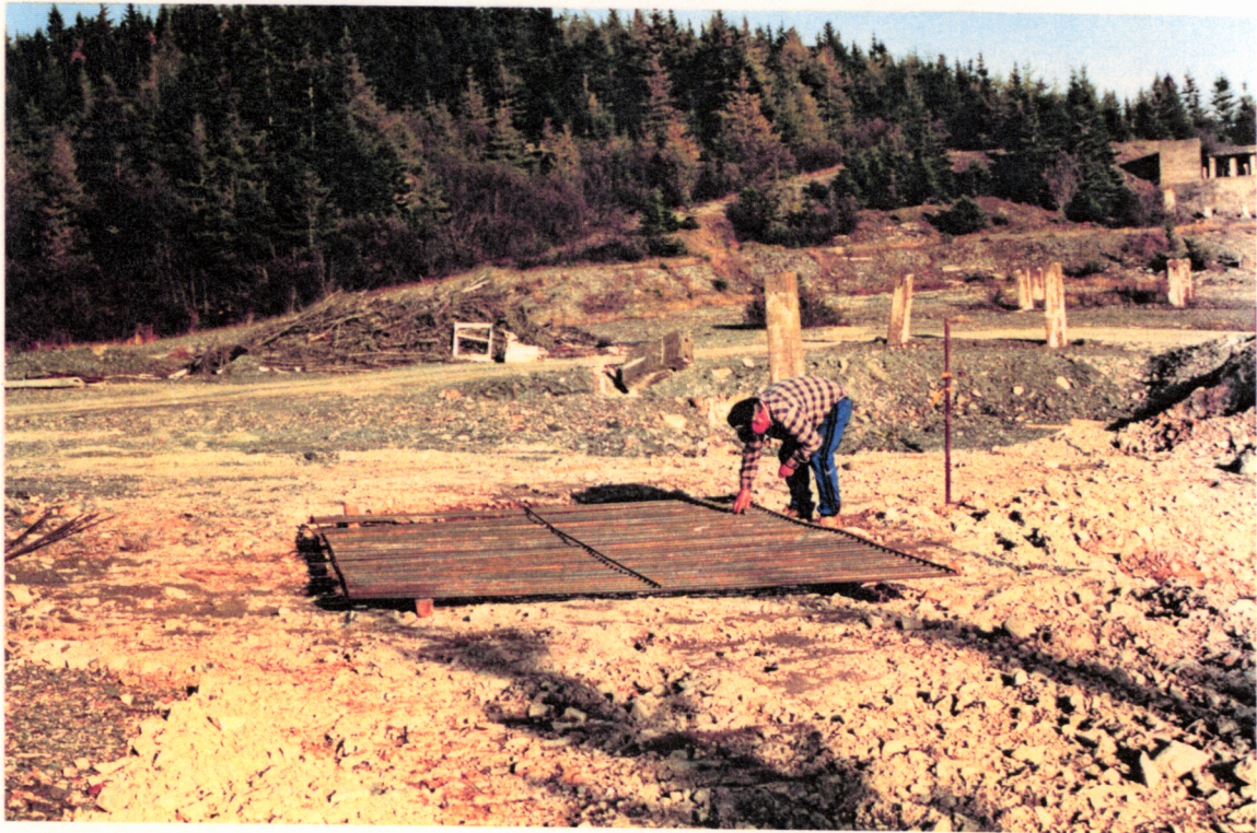
PHOTO NO. F-4: Assembling rebar mat for No. 1 Raise monolithic concrete slab.
