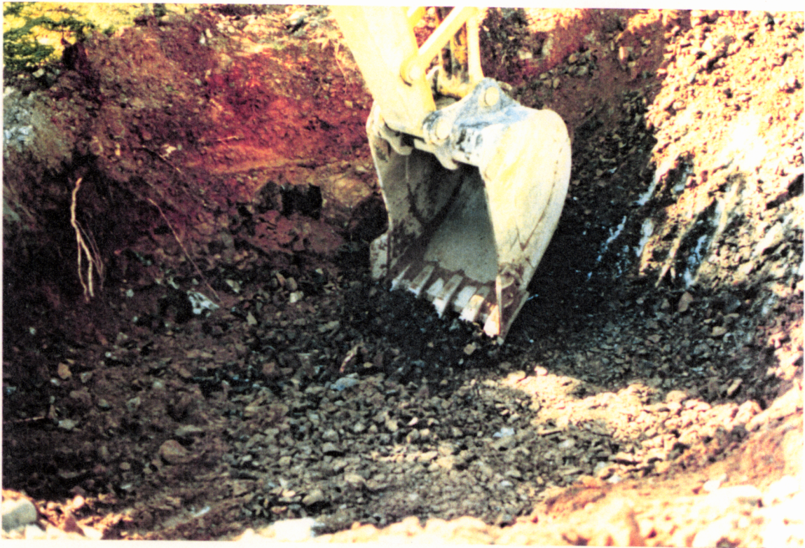
PHOTO NO. F-3: Grooming slopes and levelling base of No. 1 Raise subsidence feature.
