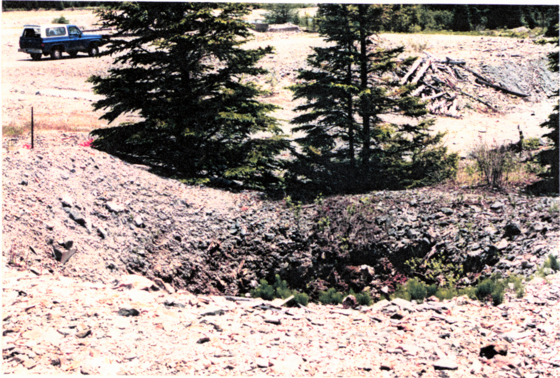
PHOTO NO. F-1: View of subsidence feature associated with No. 1 Raise.
