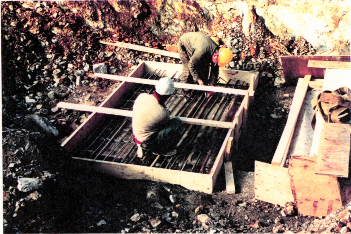
PHOTO NO. G-15: Positioning and tying rebar reinforcement in formwork of cast-in-place concrete cap.
