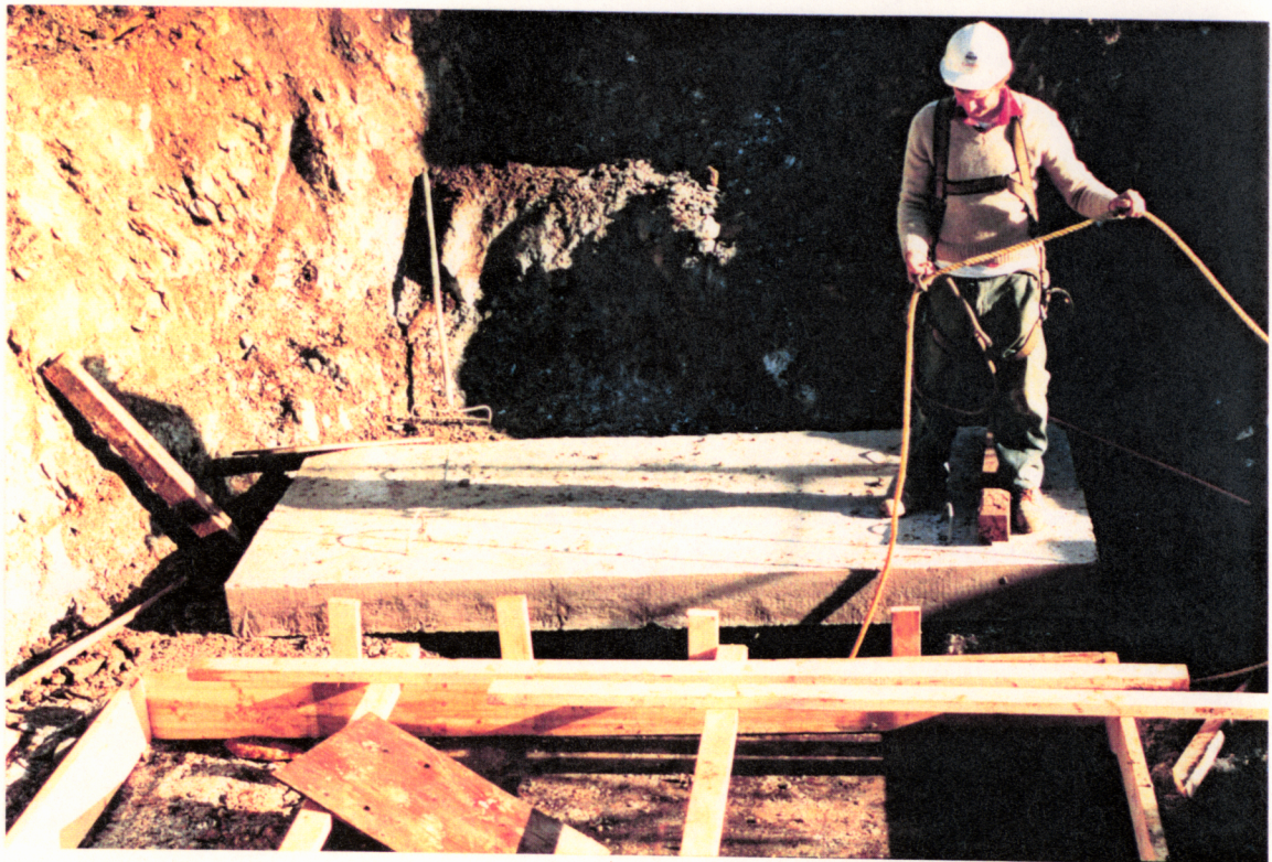
PHOTO NO. G-12: Two pre-cast panels in final location over north half of No. 2 Raise.
