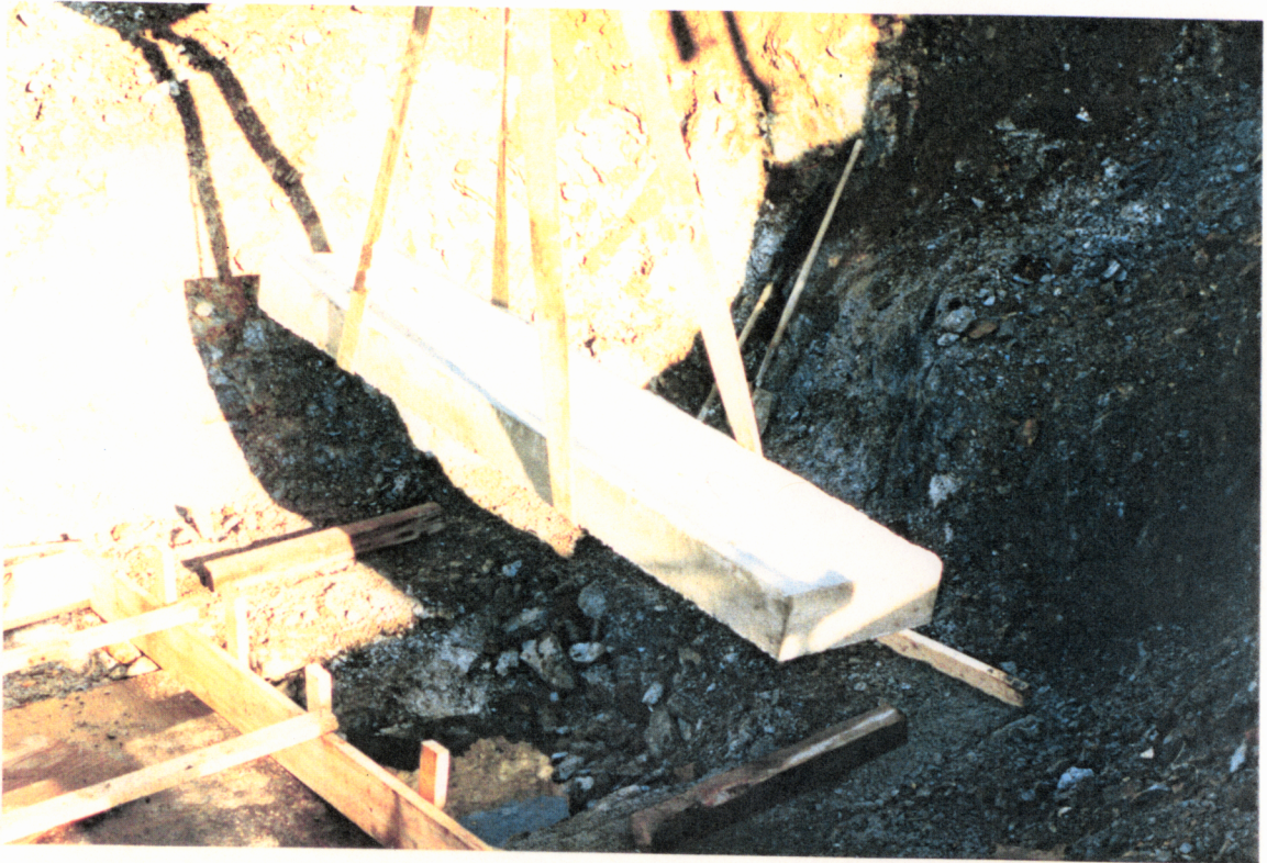
PHOTO NO. G-11: Lowering pre-cast panel onto support timbers prior to final positioning.
