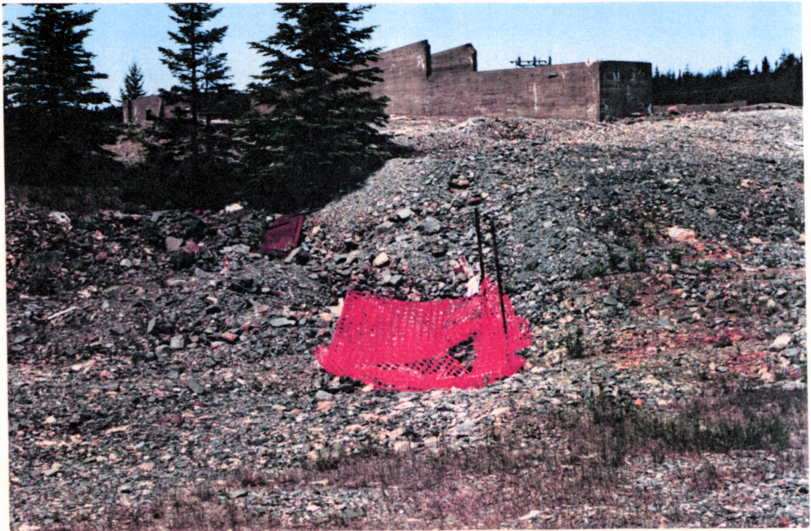
PHOTO NO. G-1: No. 2 Raise with protective barrier prior to closure.
