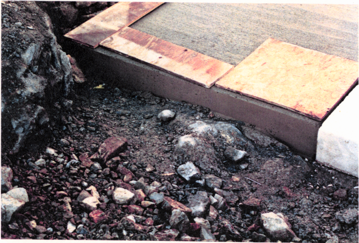
PHOTO NO. G-20: Close-up of cast-in-place concrete cap positioned on bedrock.
