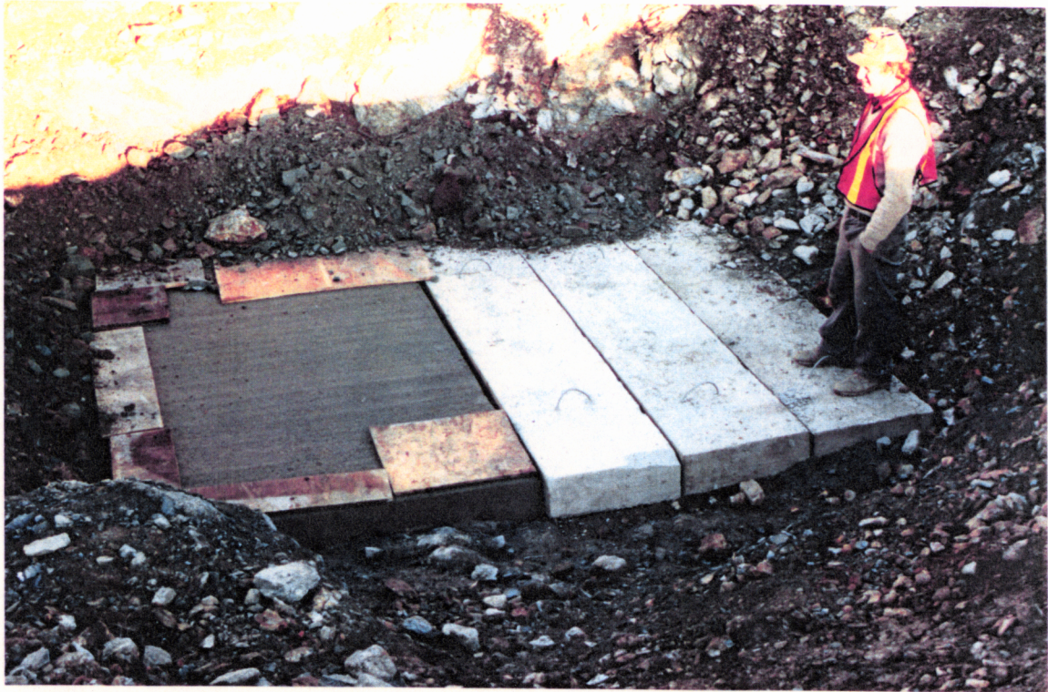
PHOTO NO. G-19: Completed cap with third pre-cast panel in position.
