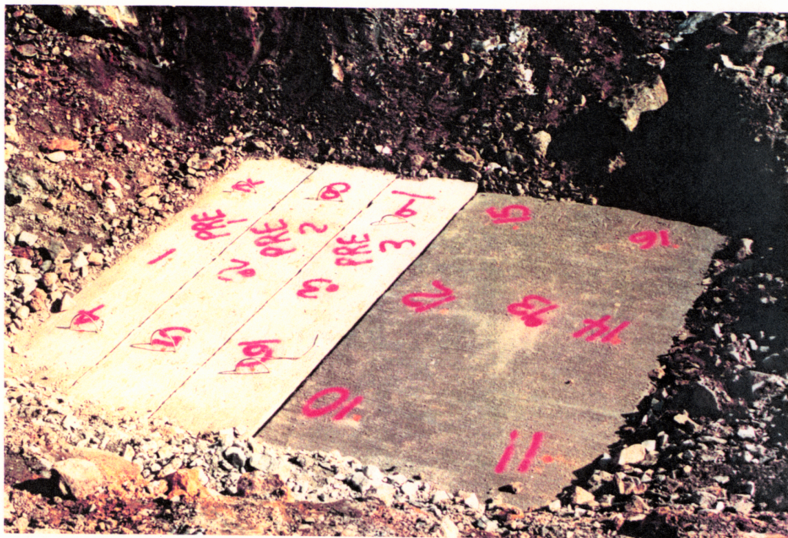
PHOTO NO. G-21: Completed pre-cast and cast-in-place concrete closure cap over No. 2 Raise with survey locations painted on concrete.
