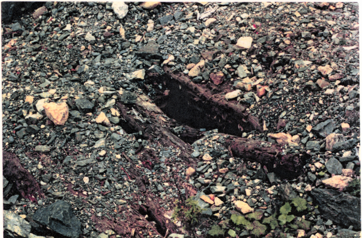
PHOTO NO. G-2: No. 2 Raise showing deteriorating timber cover.
