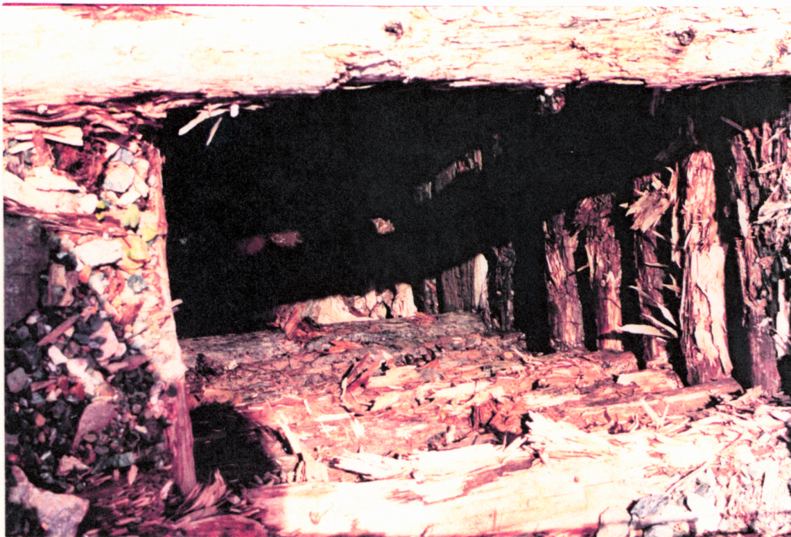
PHOTO NO. G-3: Timber lining in No. 2 Raise extending to bedrock.
