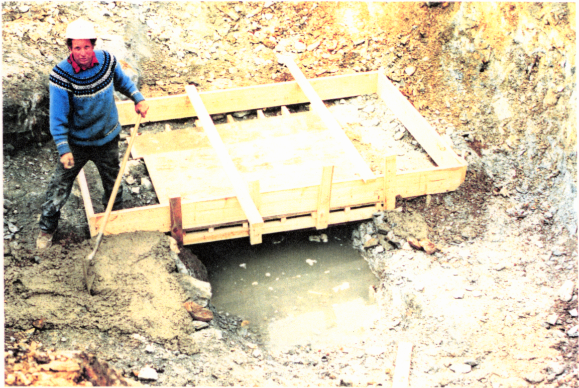
PHOTO NO. G-9: Completed formwork for cast-in-place concrete cap and spreading concrete levelling course for pre-cast panels.
