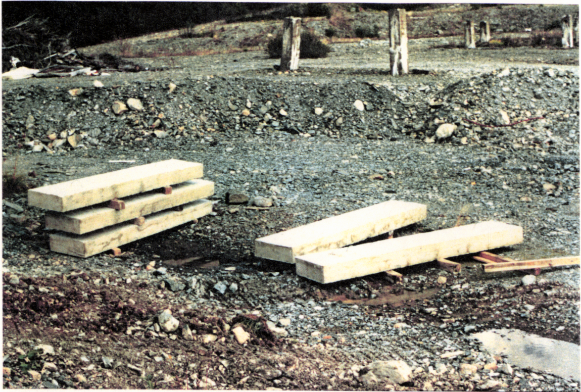
PHOTO NO. G-7: Precast panels awaiting installation with cracked panels on right.
