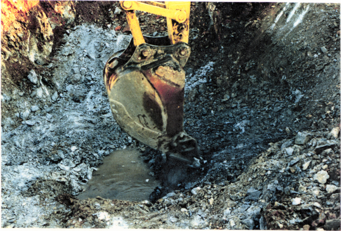
PHOTO NO. G-5: Removing loose and weathered bedrock around perimeter of No. 2 Raise.
