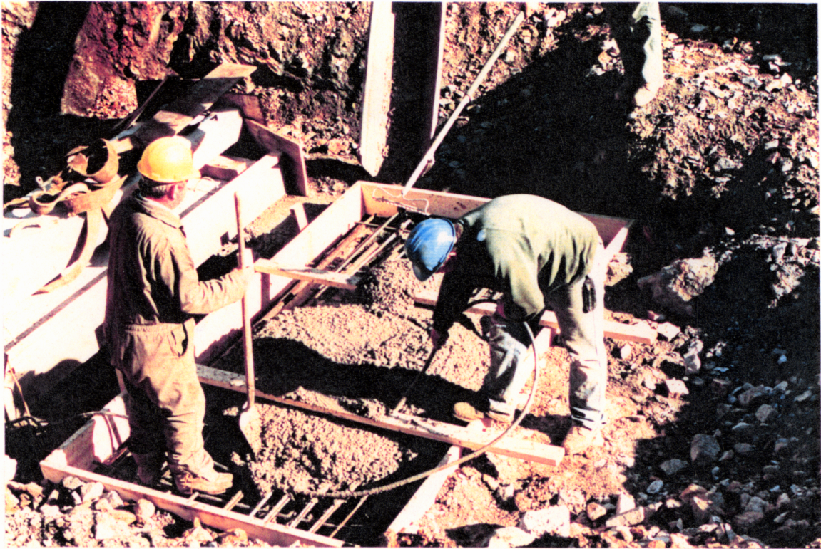
PHOTO NO. G-17: Vibrating concrete under and around rebar reinforcing rods.
