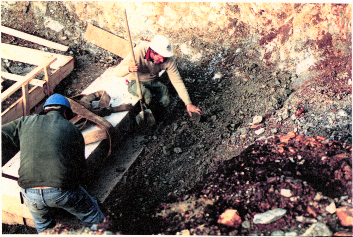
PHOTO NO. G-14: Placing well graded rock fill around pre-cast panels.
