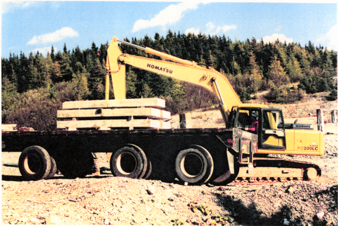
PHOTO NO. G-6: Preparing to unload precast concrete panels from flatbed.
