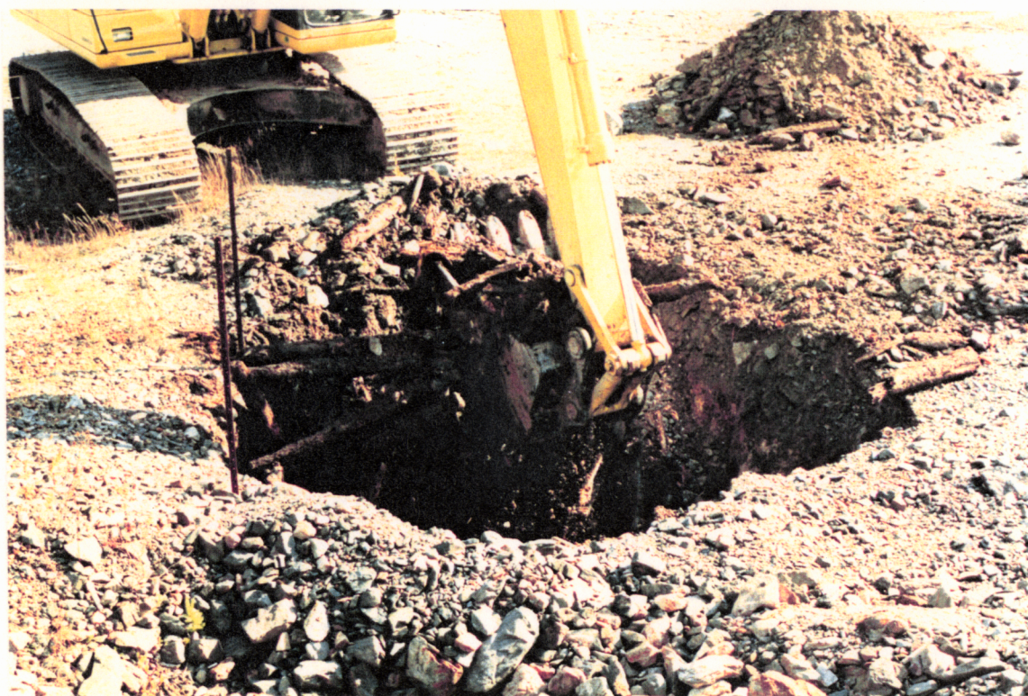
PHOTO NO. G-4: Excavating fill and timber lining around No. 2 Raise.
