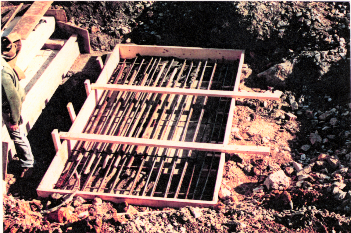
PHOTO NO. G-16: Completed rebar reinforcement prior to delivery of concrete.
