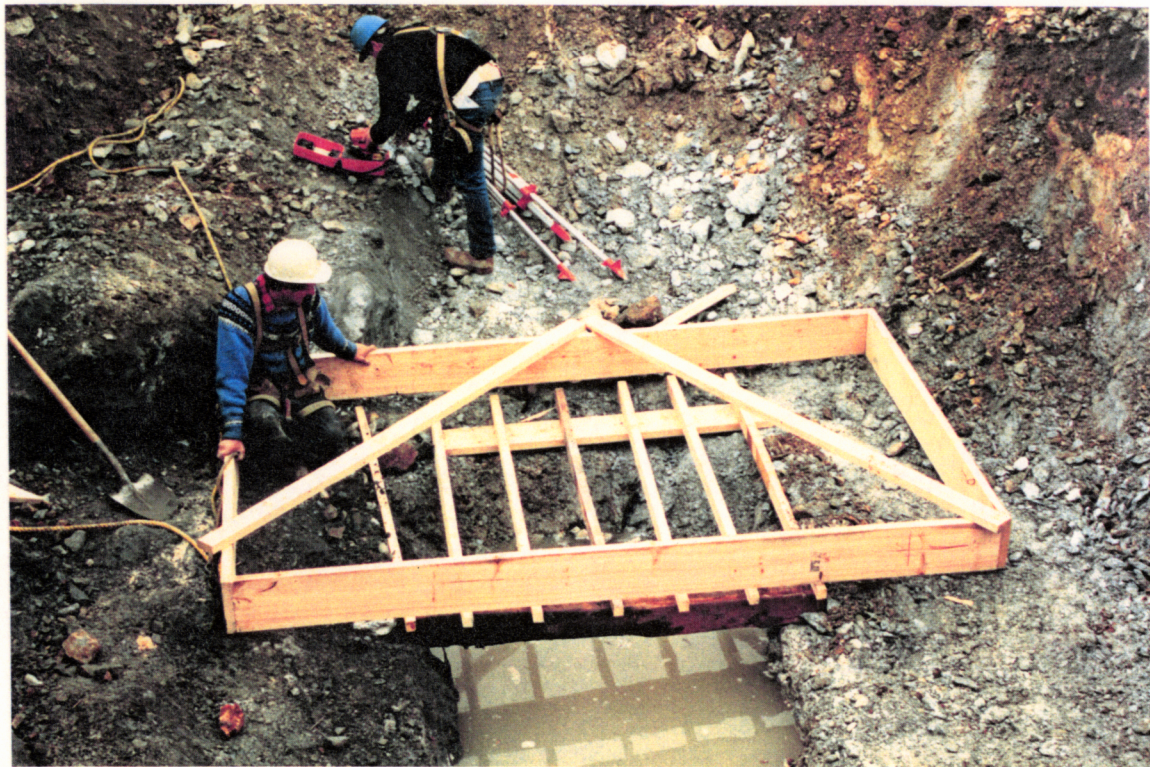
PHOTO NO. G-8: Installing formwork for concrete cast-in-place cap over south half of No. 2 Raise.
