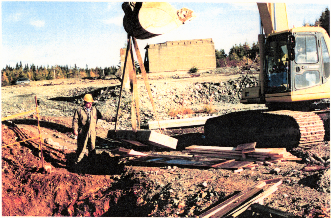
PHOTO NO. G-10: Lowering pre-cast panel into No. 2 Raise excavation.
