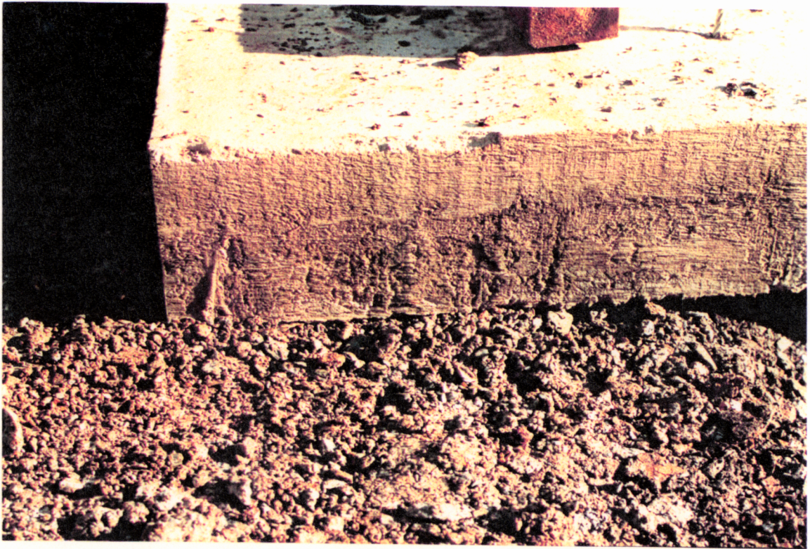
PHOTO NO. G-13: Close-up of fine rock fill levelling course under pre-cast panel.
