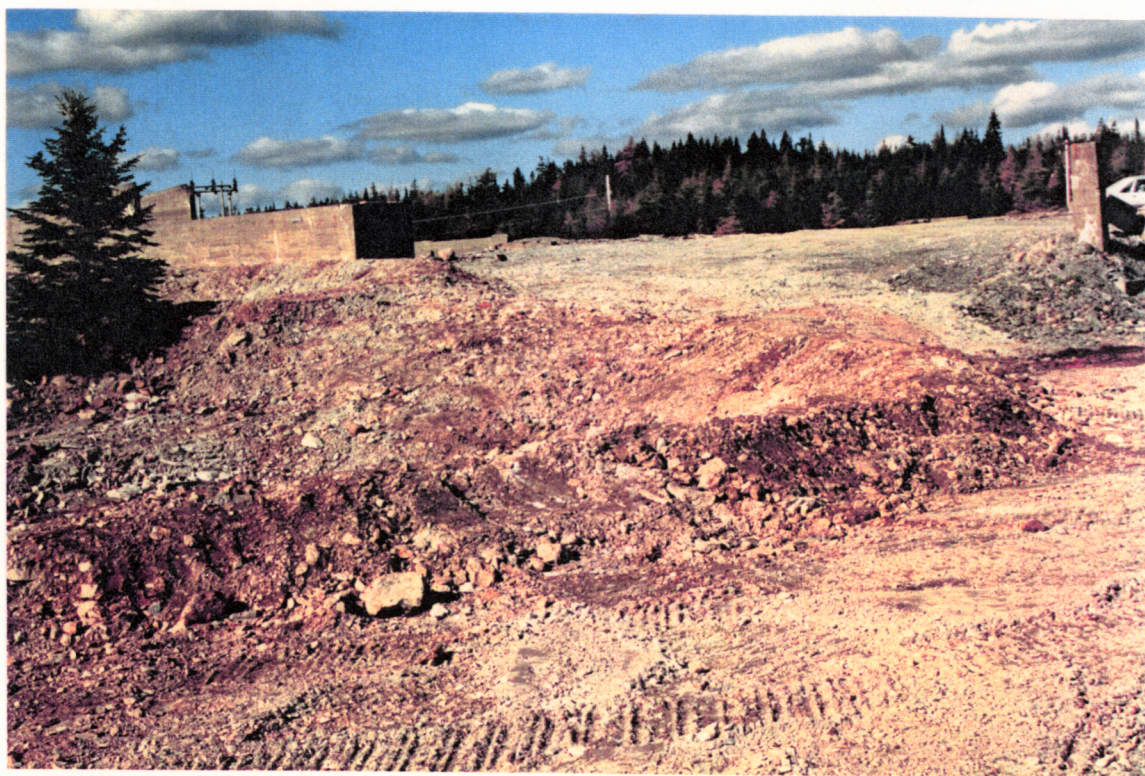
PHOTO NO. H-2: Safety berms constructed around No. 1 and No. 2 Raises.
