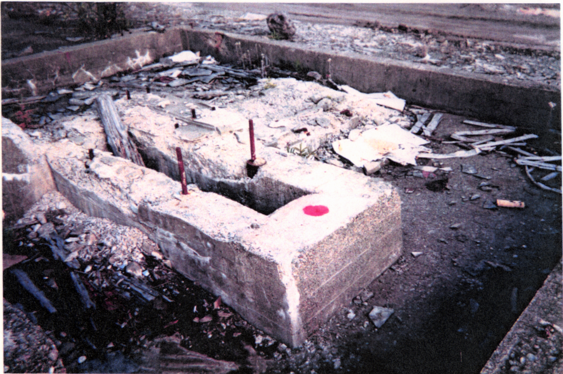
PHOTO No. H-4: Bolt in hoist room foundation used as reference elevation.
