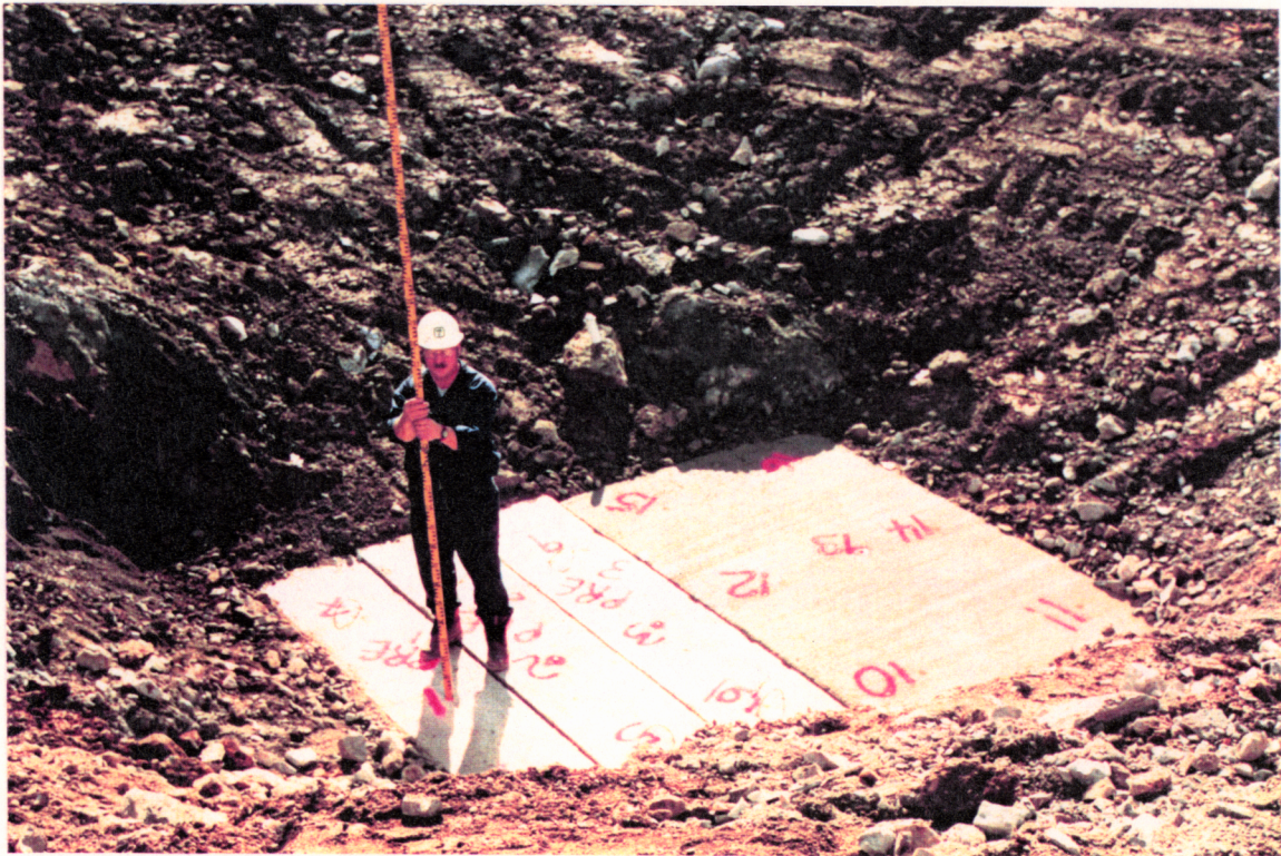
PHOTO NO. H-6: Obtaining elevations of pre-cast concrete panels and cast-in-place concrete cap over No. 2 Raise.
