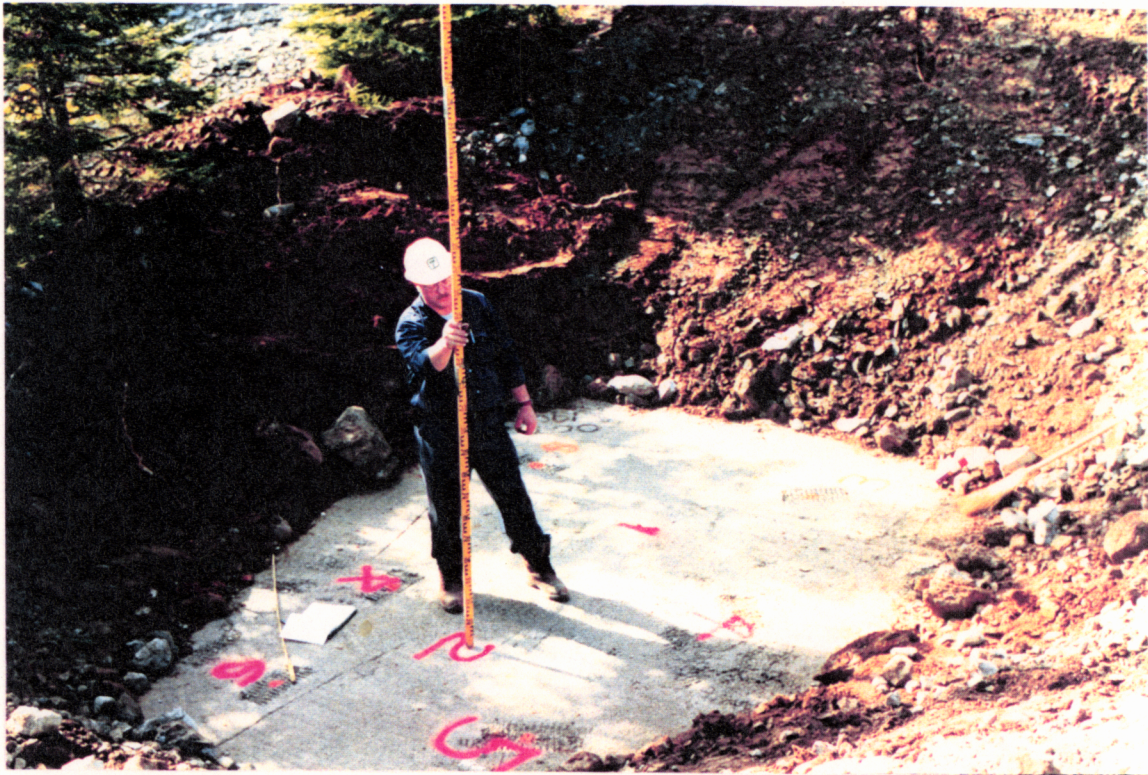
PHOTO NO. H-5: Obtaining elevations of monolithic concrete slab over No. 1 Raise.
