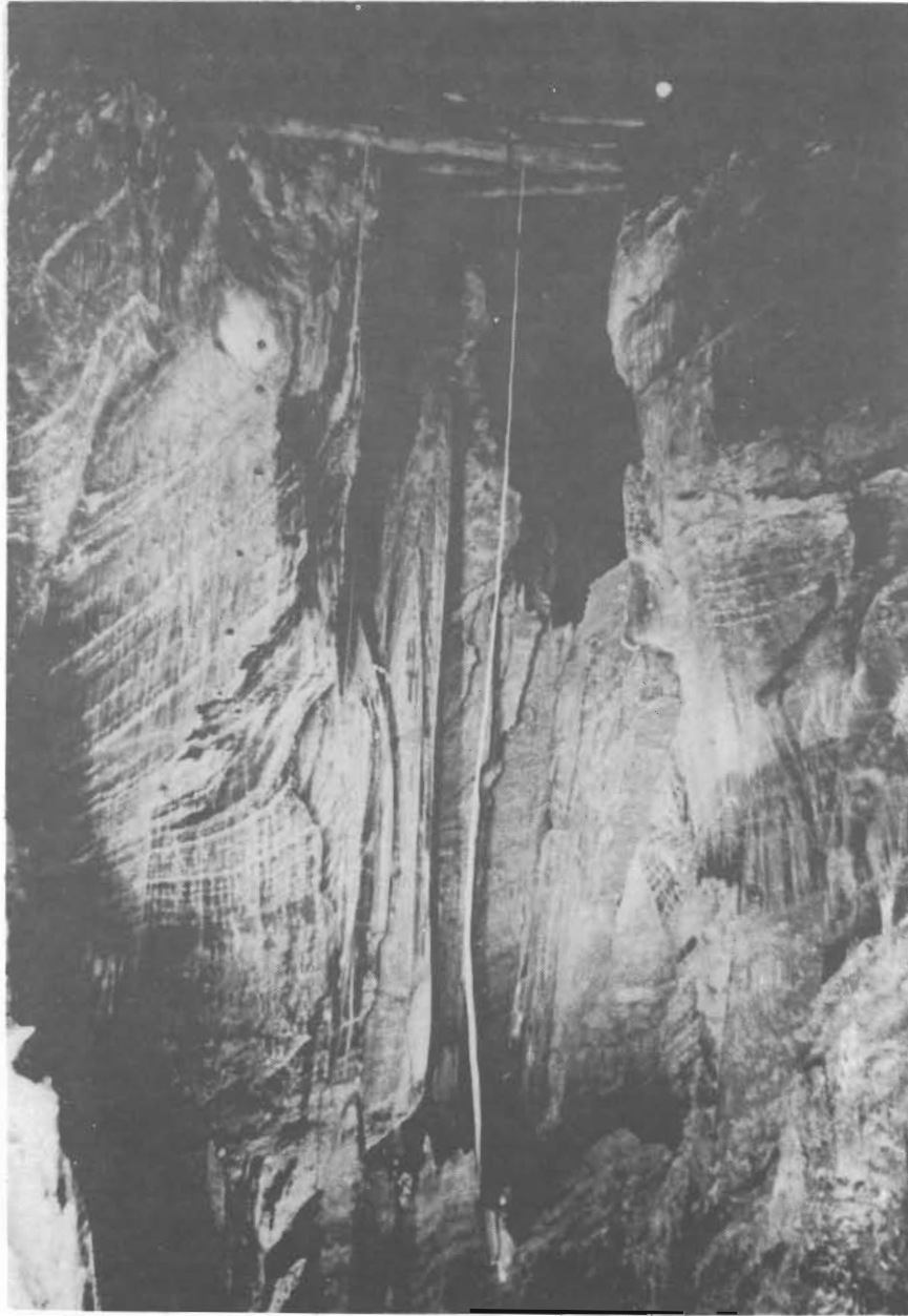
Solution mining stope after brine was pumped out in Malagash Mine. Note the relief on the rock surfaces produced by the different solubility of the salt layers.
