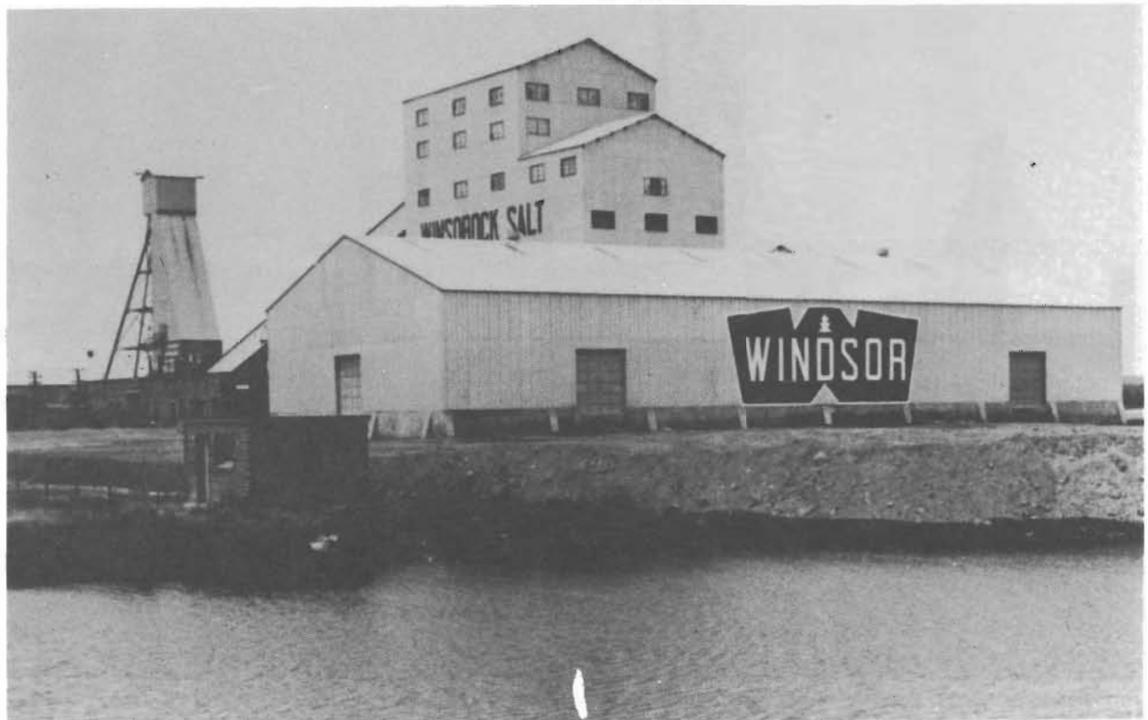
No. 1 shaft head frame and processing buildings, Pugwash Mine (NSIS).
