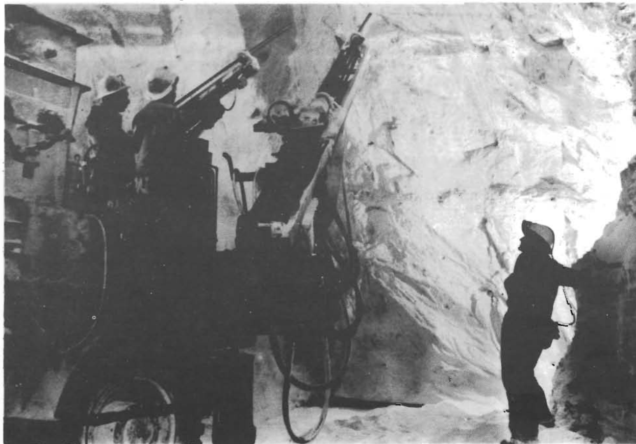
Drill used to drill blast holes in mining face, Pugwash Mine (NSIS).
