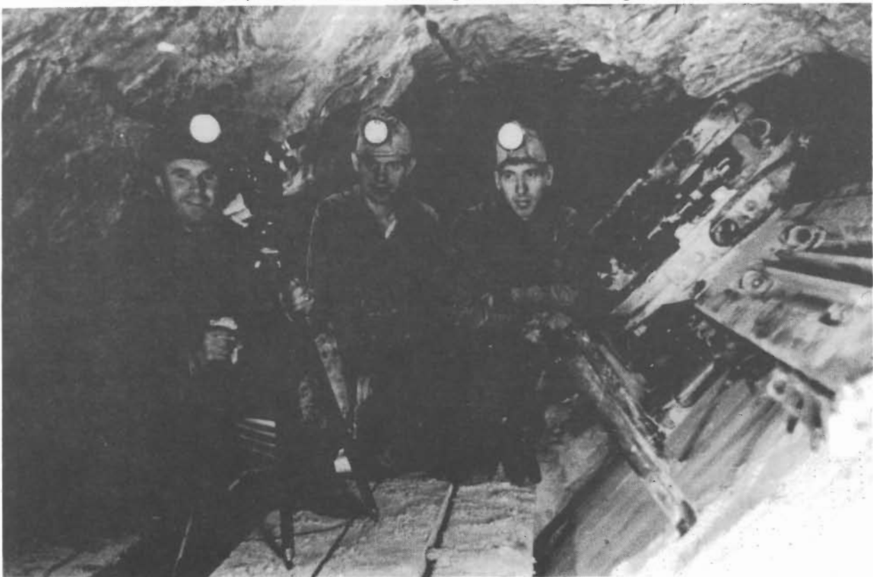
Undercutting a mine face (slope and level unknown) Malagash Mine (courtesy Reid Picture and Equipment Service),
