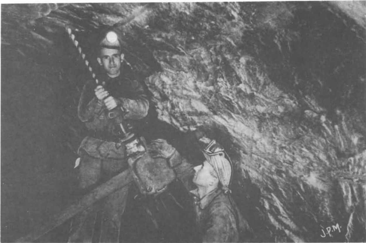
Drill setup used to drill blasting holes in the Malagash Mine.
