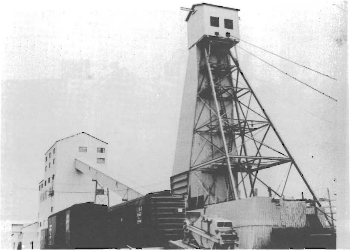
No. 1 shaft and railway loading facilities, Pugwash Mine.
