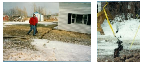
Subsidence cracking.
