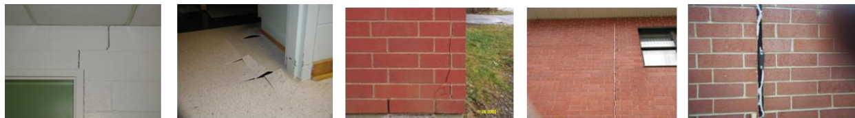
Photo 2-10 - Interior Structural Damage in a Large Structure from a Sag Subsidence Event
