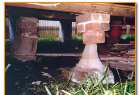
Inadequate footings ▲
