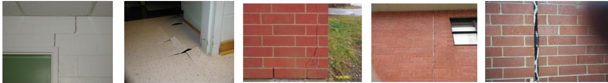
Interior structural damage in a large structure from a sag subsidence event.
