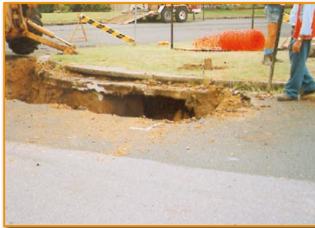
▲ Potholes from old abandoned mining are repaired by the Board where they ▼ present a public or private danger.
