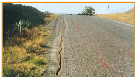
▼ The effect of tensile strains from subsidence is clearly shown on this road surface.
