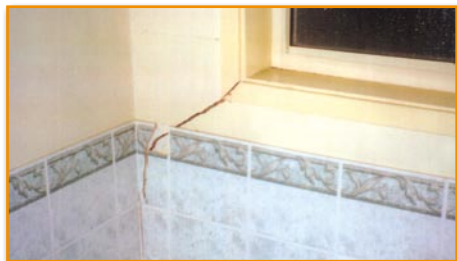
▲ Subsidence has caused internal cracking.
