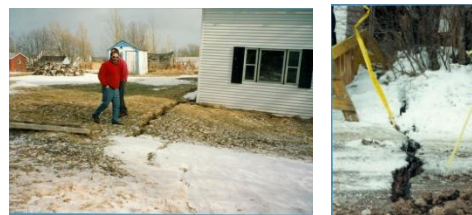
Photo 2-9 - Subsidence Cracking
