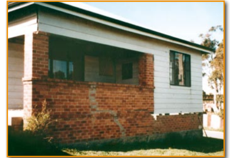
Inadequate footings ▲
