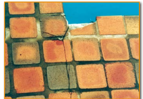
No expansion joint in pavers ▲
