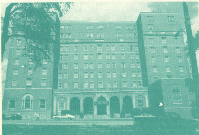
Lord Nelson Hotel. Three different types of building stone were used in the construction of this building; limestone, granite and brick (man-made from clay found in the Province).
