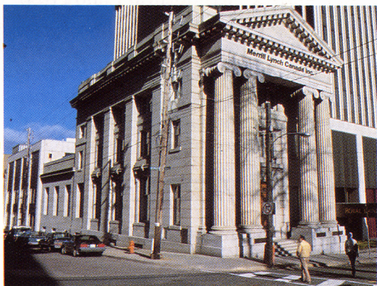
Photo 6. Merrill Lynch Building, Halifax; Terence Bay granite.
