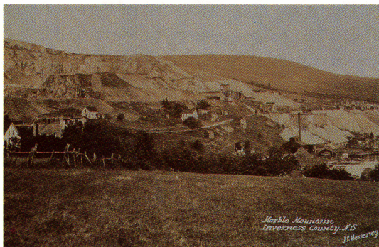
Photo 1. Marble Mountain limestone operation, circa 1920.
