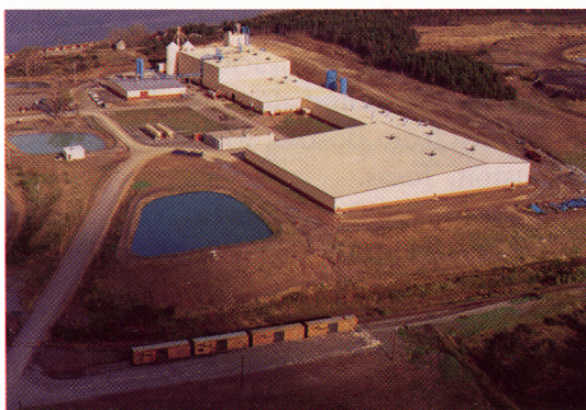
Photo 3. Louisiana-Pacific Canada Ltd.'s fibre gypsum wallboard plant at Point Tupper, Richmond County.
