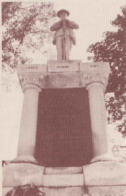
Cenotaph. The figure and columns of the memorial have been intricately carved from fine grained, grey granite. The name bearing black slabs are carved from a hard igneous rock called gabbro. (Photo: M. Devanney)
