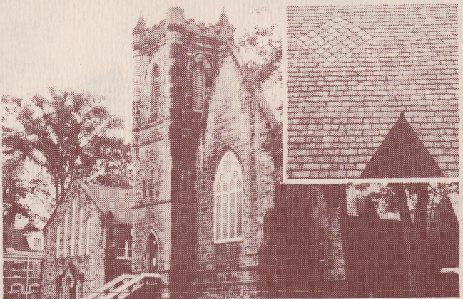
Saint John Anglican Church. The church is built from tan and pink Wallace sandstone and capped with a grey and green slate tile roof (inset). The black staining on the stone is due to air borne pollution. (Photo: B. MacBournie, Inset photo: M. Devanney)
