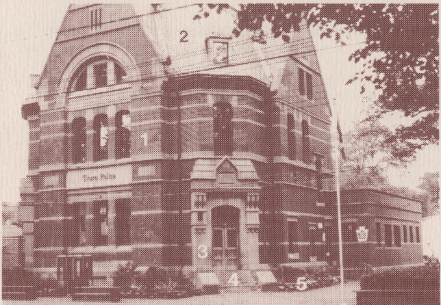
Truro Police Station. This building is composed of (1) brick made from clay, (2) slate roofing tiles, (3) sandstone and (4) granite. Blocks of slate from Wittenburg (5) surround the garden areas. (Photo: B. MacBournie)
