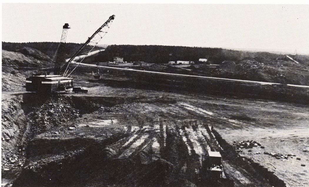
FIGURE 37. Dragline operating at the Novaco open-pit mine at Point Aconi. NSDME.
