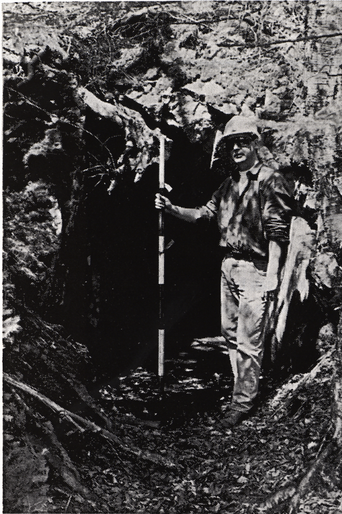
Figure 4: Adit into side of hill showing weakened and fractured rock around entrance of the opening.
