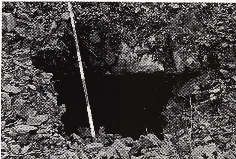
Figure 5: A mine stope extending through to surface with weak, fractured rock around the perimeter of the opening.
