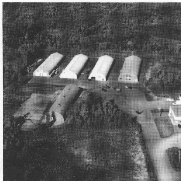
Stellarton Core Library facilities.
