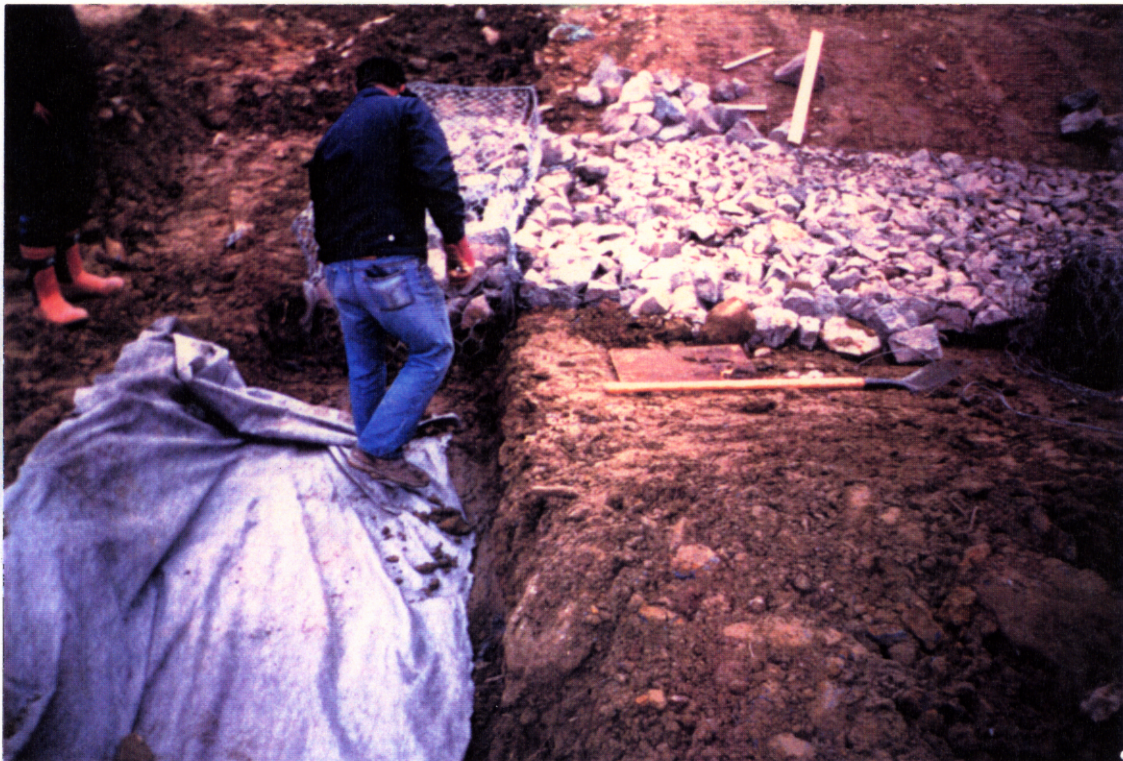
Photo #4: Construction of Spillway Intake. Gabion Baskets countersunk into existing glacial till embankment.
