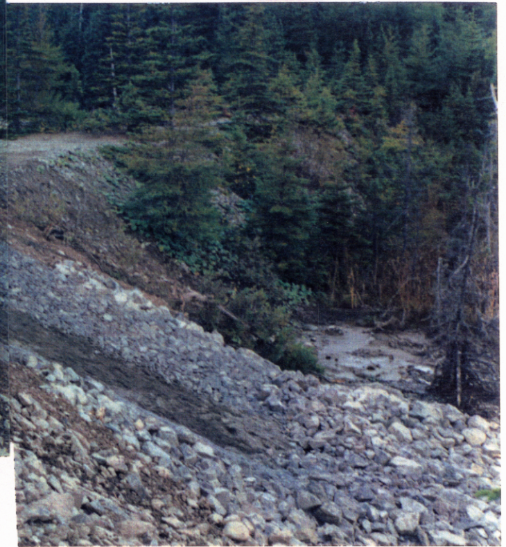
Photo #5 (above): Completed Spillway. Note ponding of water in tailings basin.
