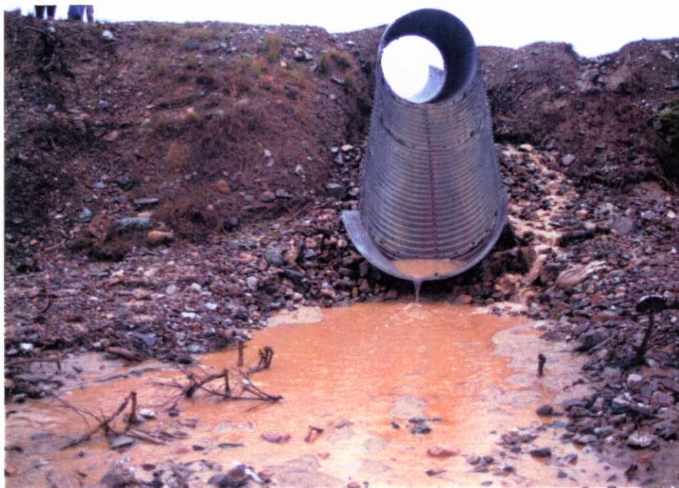
Photo #2: Discharge Outlet prior to upgrade. Note erosion and seepage to right of pipe. Sediment evident in discharge flow.
