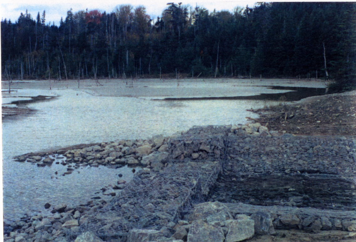
Photo #5 (above): Completed Spillway. Note ponding of water in tailings basin.
