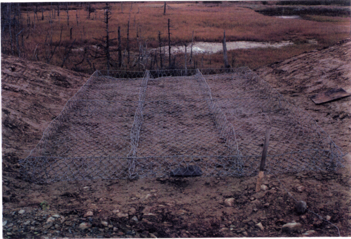
Photo #3: Gabion Mattresses placed on heavily compacted glacial till berm. Sand placed latter to provide cushion/filter with rockfill.
