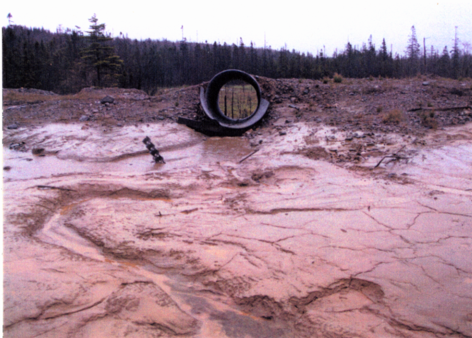
Photo #1: Discharge Structure Intake prior to upgrade. Note runoff water flowing under culvert.
