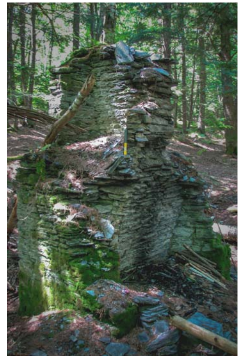
Figure 2. Remnants of the fireplace of the two-storey manager's house at the Sibley Mountain slate quarry; rock hammer for scale.
